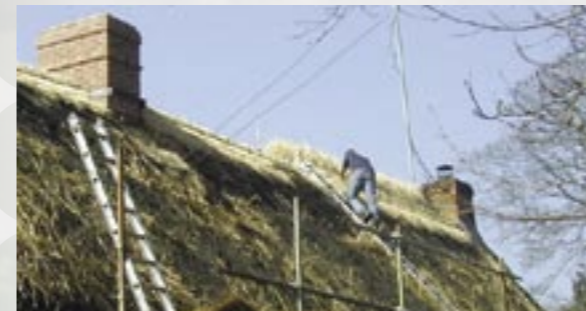
Thatching in progress
