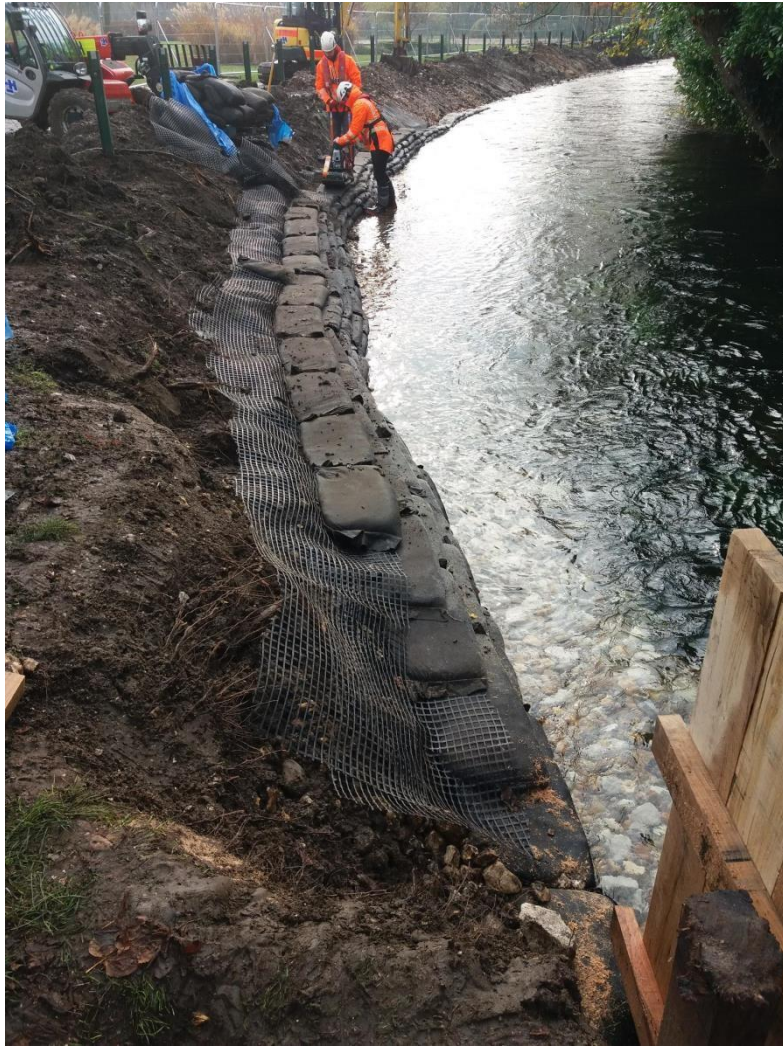
Stage 2 Revetment work on the Test
