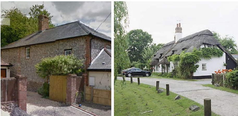
FIGS 24, 25, 26 & 27 - examples of decorative flint and brickwork, fenestration, roofing materials and boundary treatment
