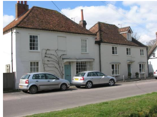
Village houses, fronting directly onto road. Painted brick walls and tiled roofs.
