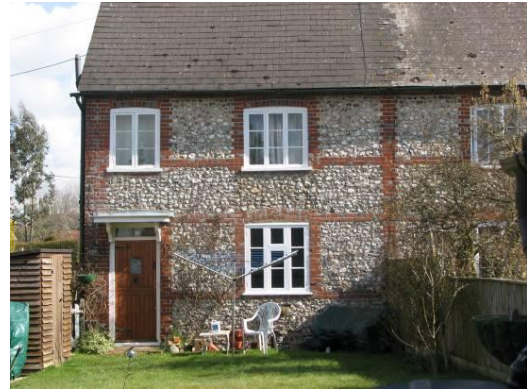
Semi detached cottage. Traditional brick and flint walls and slate roof
