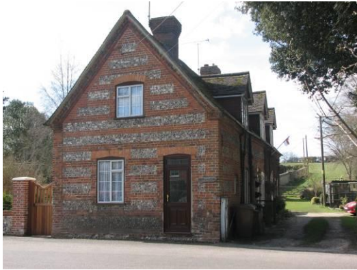
Traditional brick and flint terrace of cottages, side on to public highway
