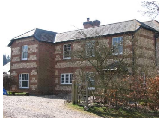
Detached house, brick and flint walls, slate roof
