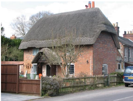
Traditional cottage. Red brick walls with thatched roof
