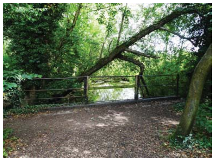
2 THE OLD RAILWAY BRIDGE OVER PILL HILL BROOK
