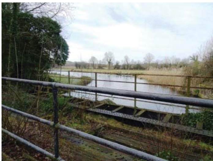
1 THE PATH USES THE DISUSED RAILWAY BRIDGE TO CROSS THE RIVER TEST AND CROSS THE CHILBOLTON AND WHERWELL PARISH BOUNDARY
