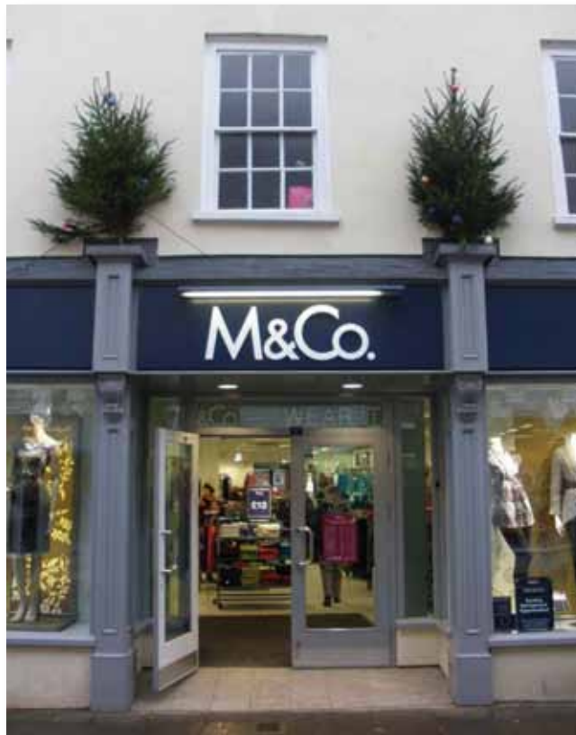
Fig. 22: 7-9 The Hundred, Romsey. Pilasters frame the entrance of this early 21st century shopfront which helps to give a vertical emphasis to the elevation.
