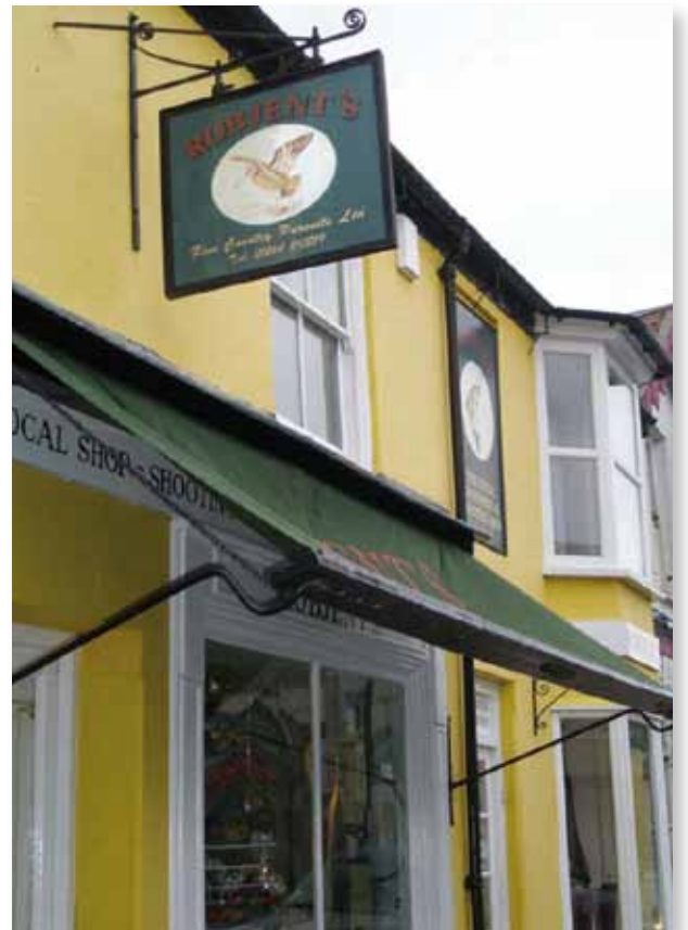
Fig 39: Traditional style canopy. High Street, Stockbridge
