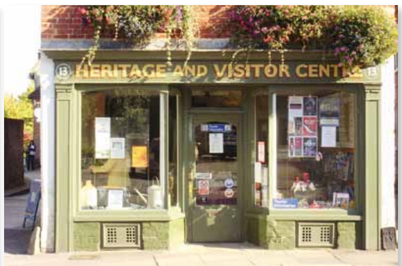
Fig. 9: Traditional brick stall riser in 19th century shopfront. Church Street, Romsey
