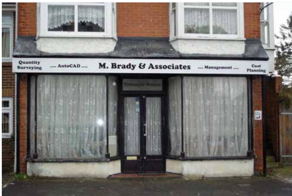
Fig. 10: Recessed doorway in late 19th century/early 20th century shopfront. Old Winton Road, Andover
