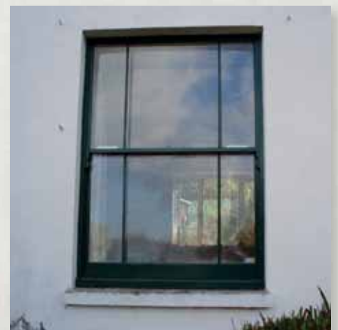
Chalkdell House sash window
