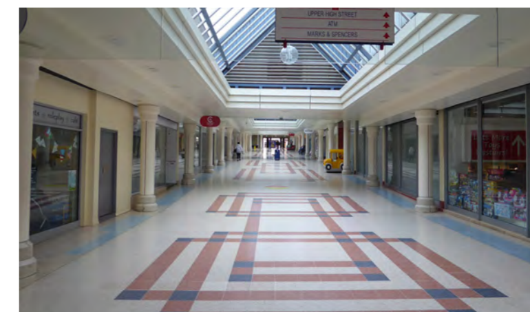
Covered roof is very low to mall floor, heavy and outdated in appearance
