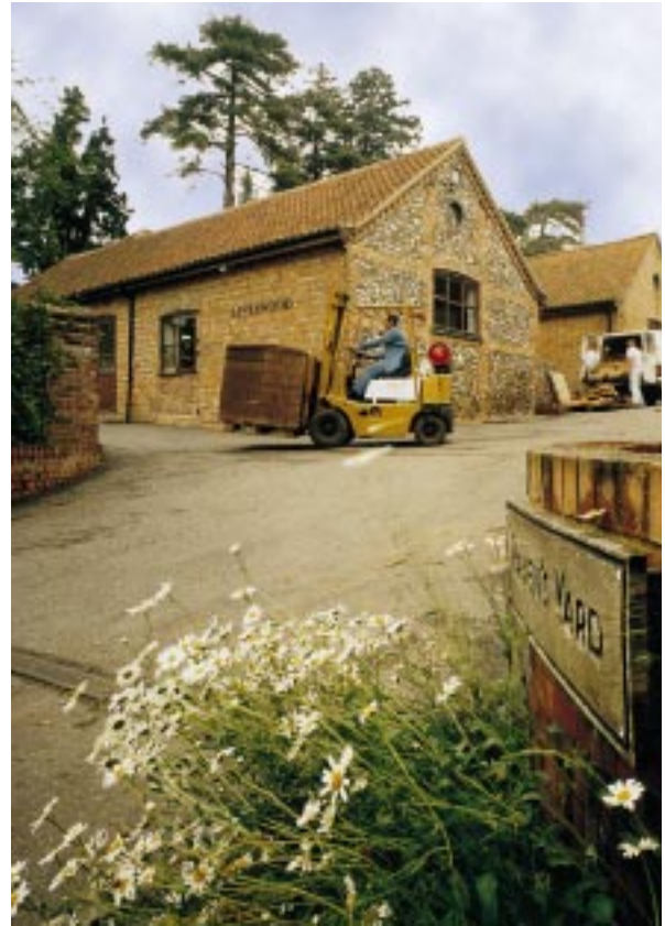
Village-based employment in new or converted buildings contributes to the future sustainability of village communities.
