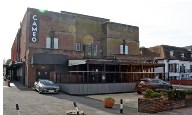
A large-scale modern building (former cinema in use as a nightclub) at the east end of London Street
