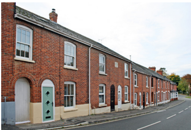
Examples of traditional windows, doors and rainwater goods being replaced with plastic versions in Marlborough Street
