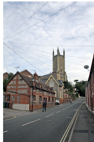
Overhead wires in Marlborough Street
