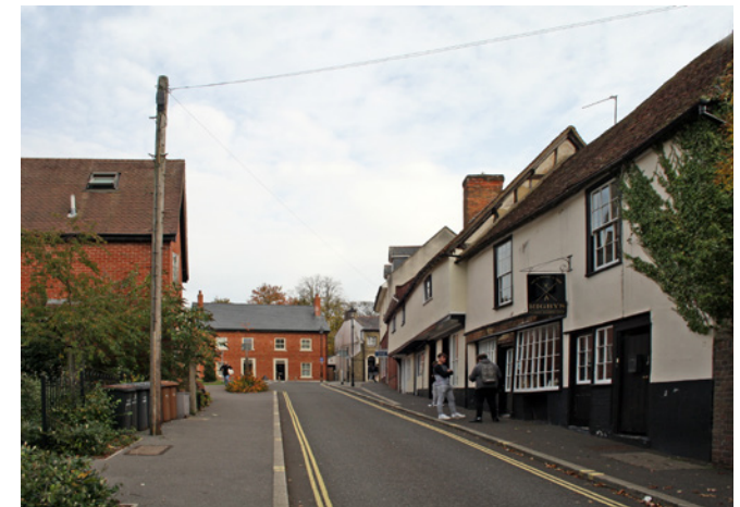
View looking east along Chantry Street showing medieval, partly refronted buildings on the right
