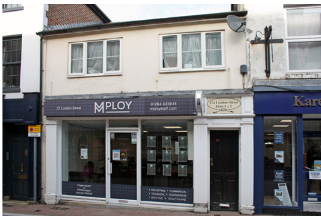
Timber windows replaced with uPVC units in London Street
