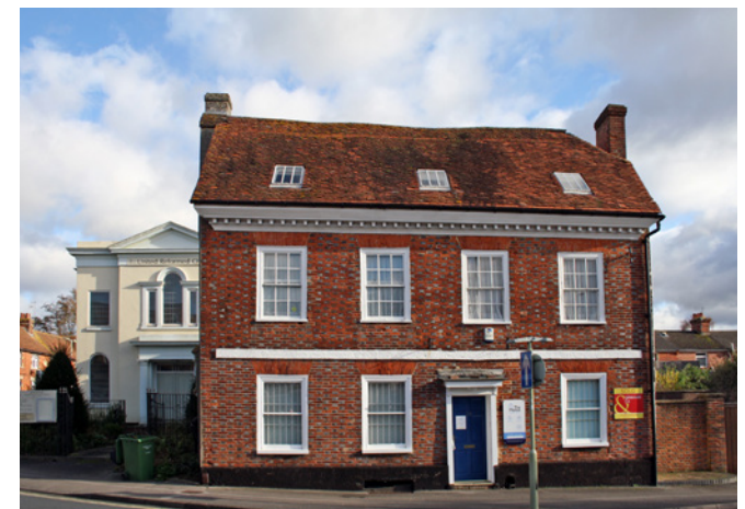
A view of the north end of the character area showing No.54 East Street on the right, the United Reformed Church in the middle and Acre Almshouses on the far left
