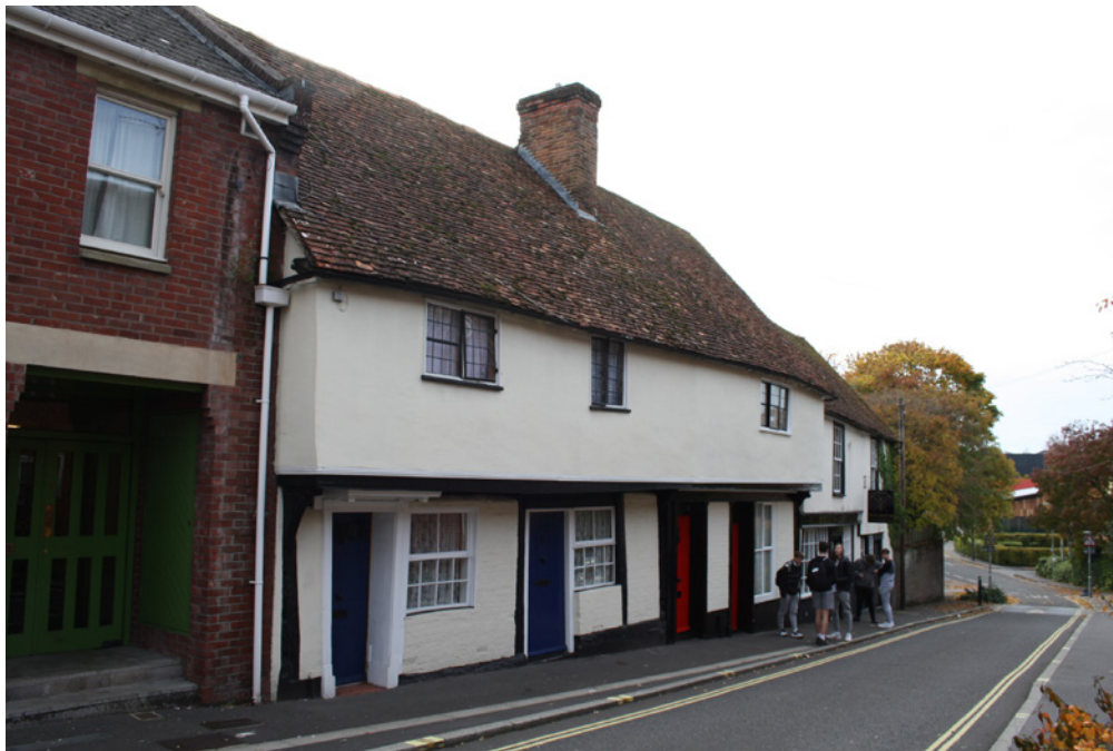
Buildings at Nos.11, 13 and 15 Chantry Street comprising 16th century fabric and subsequent alterations
