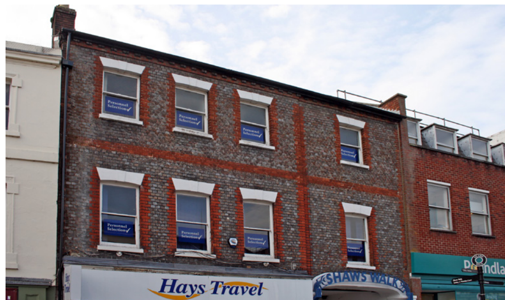
Plastic film advertising applied to upper-level windows
