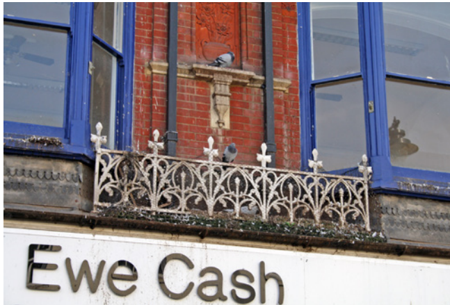
Bird roosting causing considerable build-up of guano
