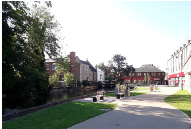
The recently upgraded public realm along the river Anton to Bridge Street.
