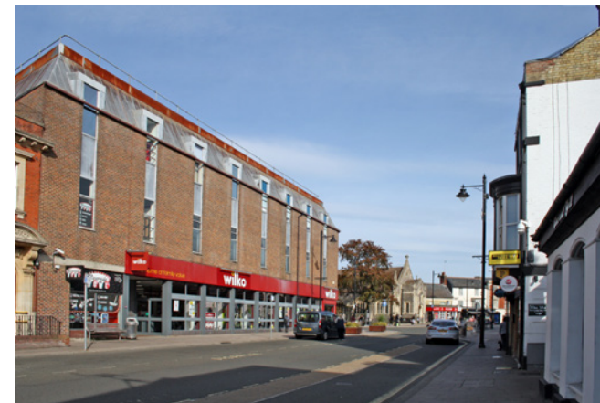
Nos.22-30 Bridge Street detracts from the special interest of the Conservation Area owing to its oversized scale, unsympathetic materials and detailing
