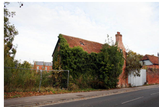
The Anton Laundry is a Grade II listed building which is suffering extreme decay
