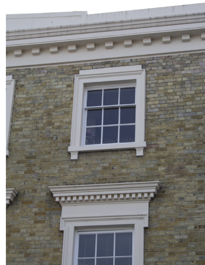
Decorative features including dentilled or bracketed cornices and rendered window surrounds
