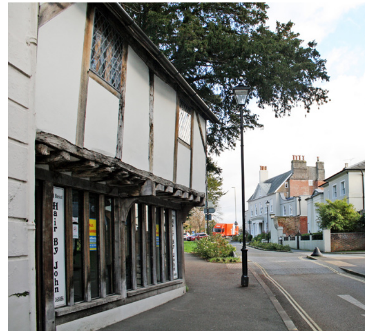
Timber-framed, jettied building dating to the 17th century at 84a High Street
