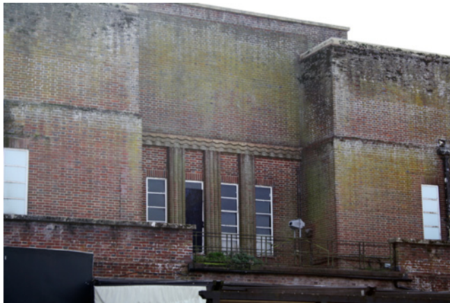
Foliage and algae growth to elevation of the former cinema in London Street
