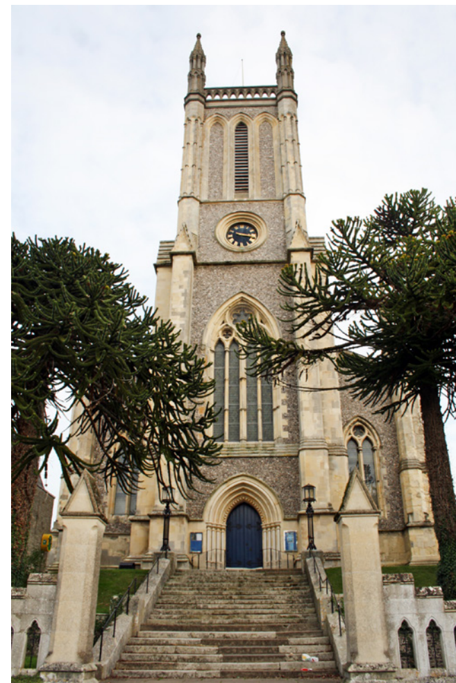
View of the west elevation of St Mary's Church showing the prominent tower
