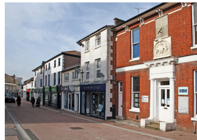
Terraced buildings along the north side of London Street (west end)
