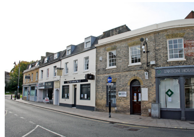
Terraced houses at the north end of Winchester Street
