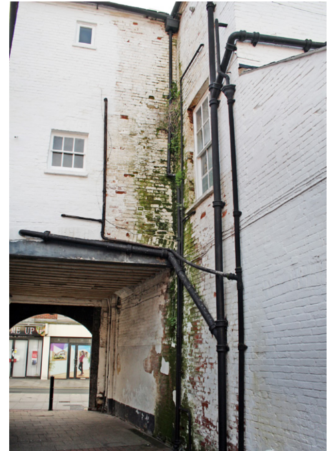
Broken rainwater goods causing damage in Waterloo Court
