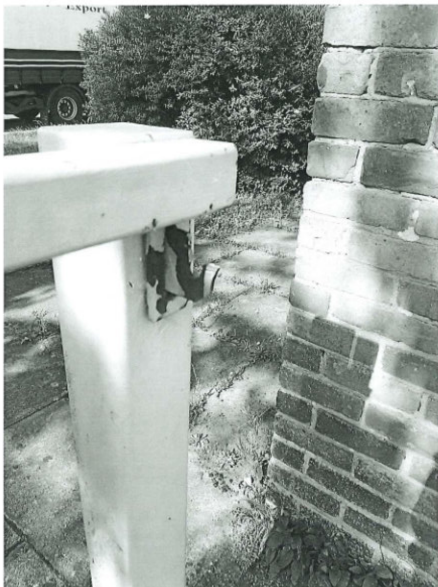
Picture showing damage to lock
