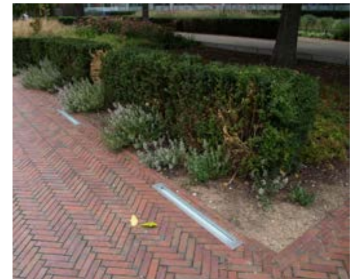
Clay Pavers and Edging to Public Footway / Moulded edge, 85mm wide x 200mm.
