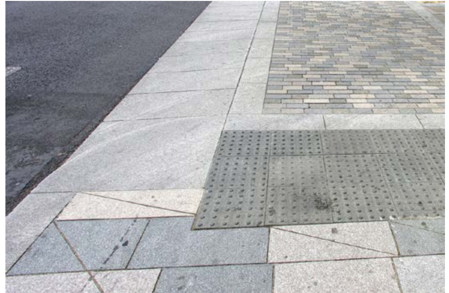
Good side street detailing / Sidcup
