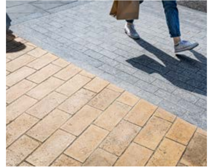
Use of Purbeck limestone setts / to announce a threshold between the high street and a narrow yard as shown along Borough High Street, London.
