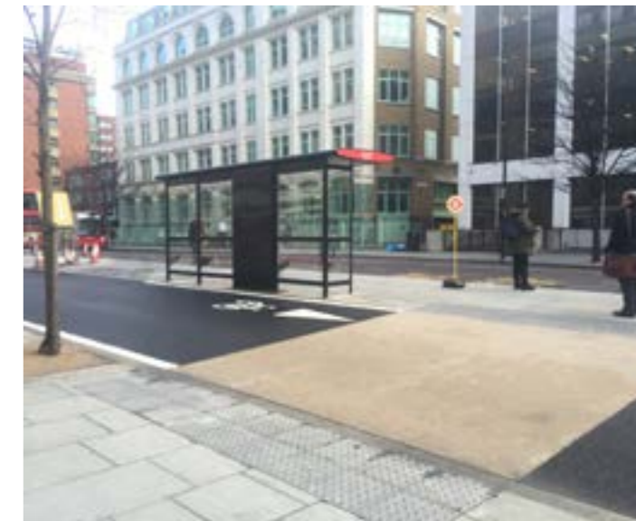
Asphalt Cycle Track / Clearly identifiable as a movement corridor with buff pedestrian crossing
