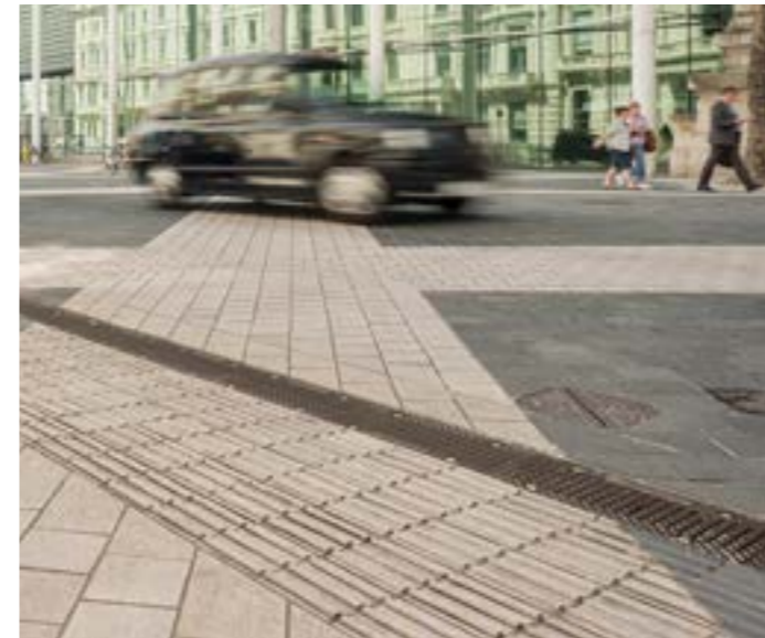
Heavy duty channel drain with cast iron cover / draining both carriageway and footway. 'Birco' type heavy duty channel drain from Marshalls with slotted cast iron cover. Care should be taken to specify heel and slip resistant finishes, Exhibition Road, London
