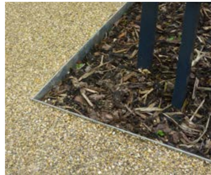
Beige Mix Resin Bound Gravel / Monolithic poured material.
