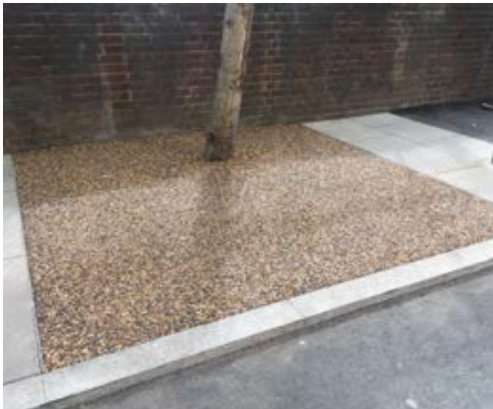
Resin bound gravel / finish to treepits where existing tree root protection areas are important in inner 'Town' areas.
