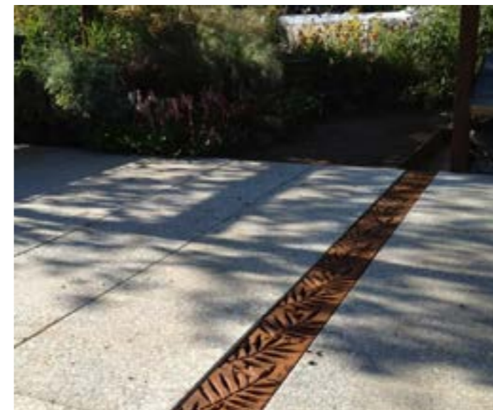
Decorative cast iron cover / channel drain cover in footway directing surface water to planted area. Iron Age Grates
