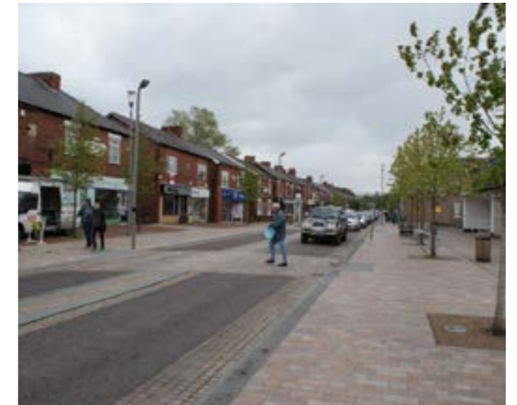
Extended kerbside channel / using 6 rows of small setts directs water flow and encourage responsible driving. In Poynton
