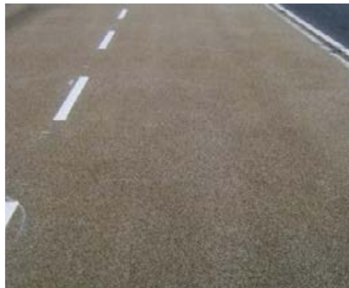
Hi-friction slip resistant resin bonded aggregate / applied to wearing course provides a lighter surface and helps prevent traffic accidents.
