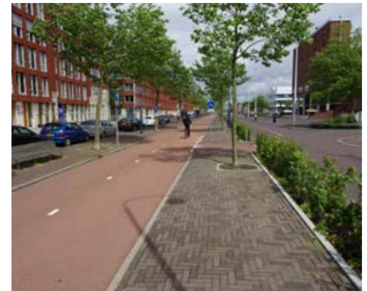
Coloured Asphalt Cycleway and Clay Paver Footway / Monolithic poured material with clay pavers.
