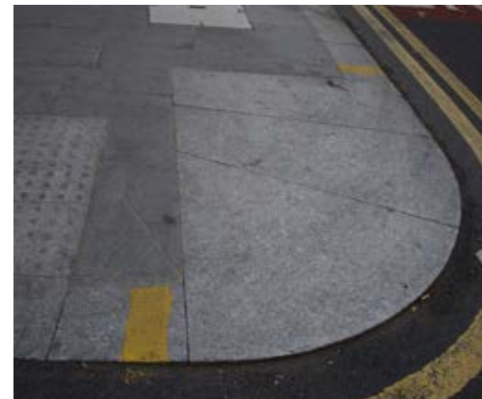
Granite quadrants and 'specials' / improve appearance of kerbline at junctions. Example: Leyton High Road
