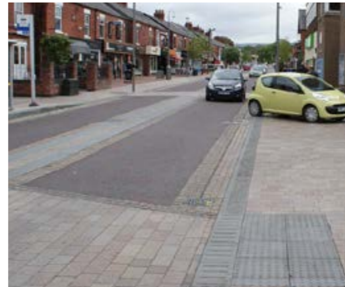
Median strip in natural stone / separates carriageways and minimizes area of asphalt in Poynton.
