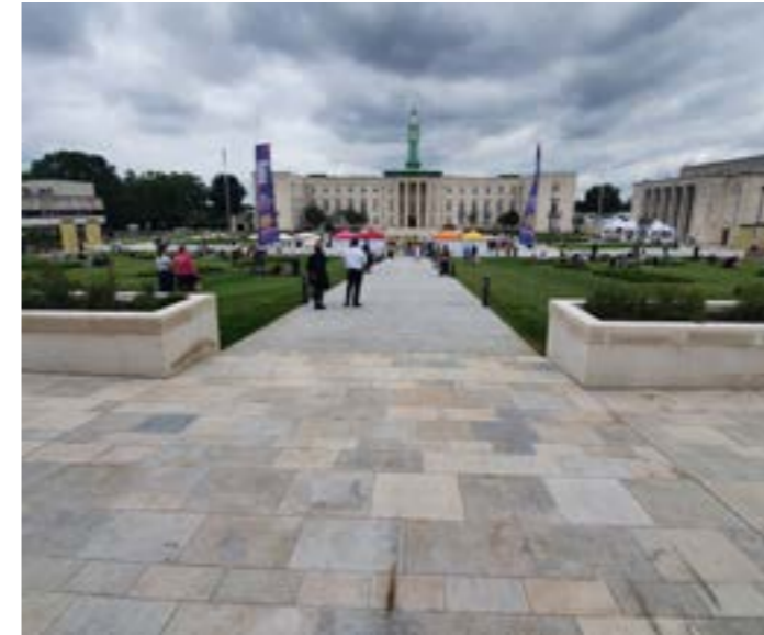
Public Spaces / Limestone as high quality highlight material to key public space features, eg Lower High Street 'runner'.
