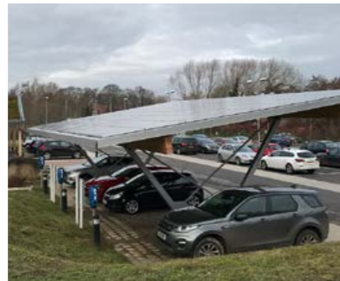
Charging within car parks, using solar
