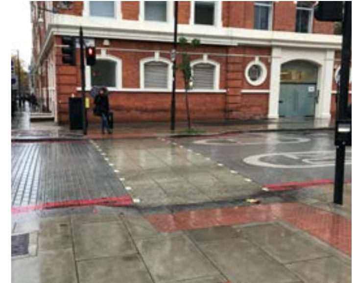
Concrete imprint / used at crossing to harmonise with general footway materials in the street on Camden Road, London.
