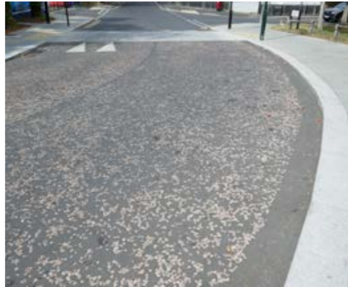
Light coloured stone aggregate / rolled into darker asphalt wearing course to improve appearance and reduce surface area of heat absorbing dark asphalt.
