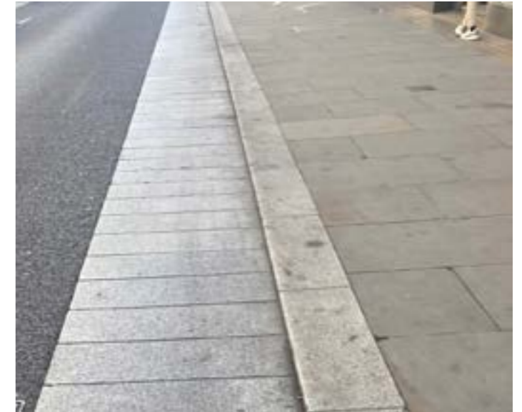
Granite kerb with extended granite channel / edge detail helps to minimise extent of asphalt in the carriageway. Example: New Bond Street, London
