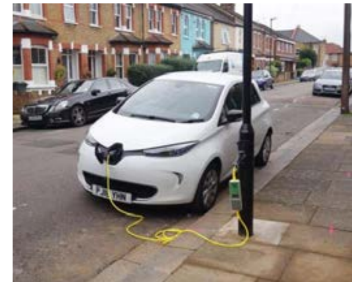
Residential lamp column charging / London
