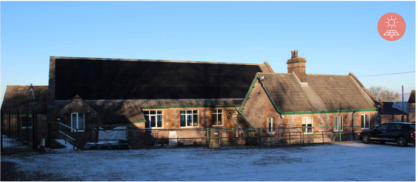
South-facing roof slope of the main hall with 60 PV panels installed
