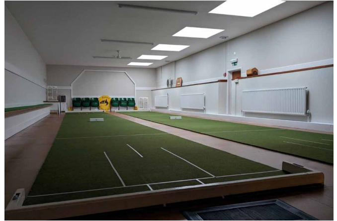
Rooflights installed above a skittle alley in Otterhampton Village Hall
