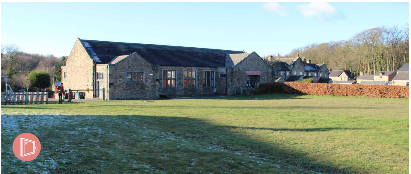
The hall benefits from a large field directly behind it, providing an ideal area for a shallow coil system, part of the ground source heat pump.
