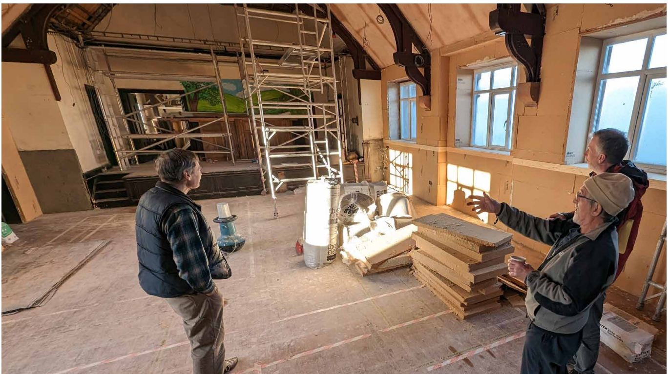
Skelton Toppin Memorial Hall during the installation of internal wall insulation
