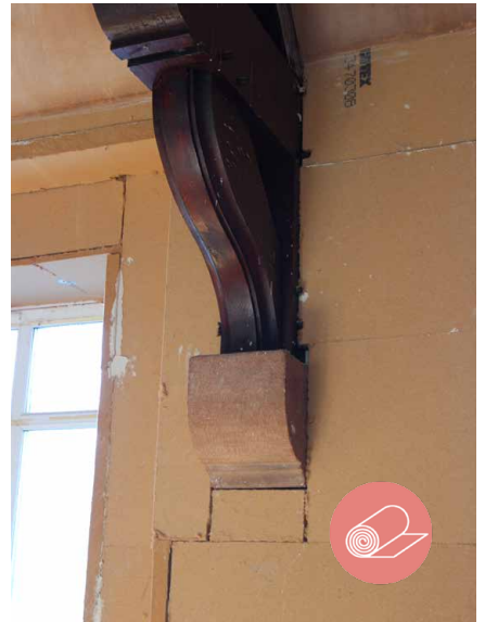
40mm breathable wood-fibre insulation panels are installed to all internal walls, co-ordinated around architectural features
