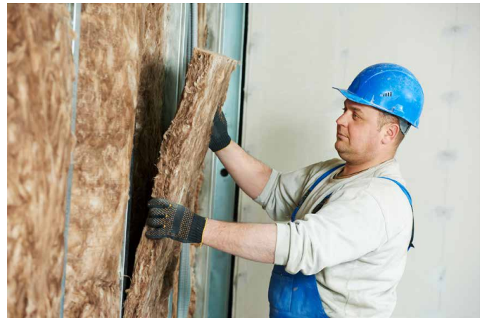
Internal wall insulation
