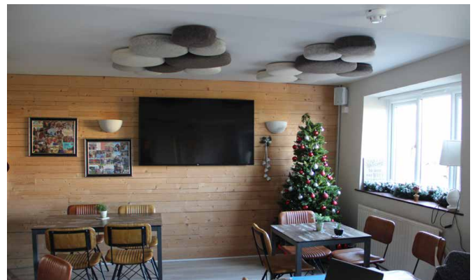
Natural acoustic ceiling cushions from The Woolly Shepherd were installed at Otterhampton to soften the acoustic
