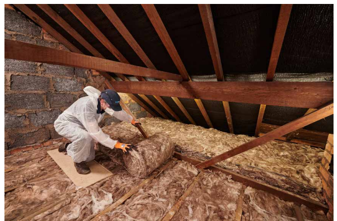
Properly installed ceiling insulation. Photo courtesy of Knauf Insulation.
