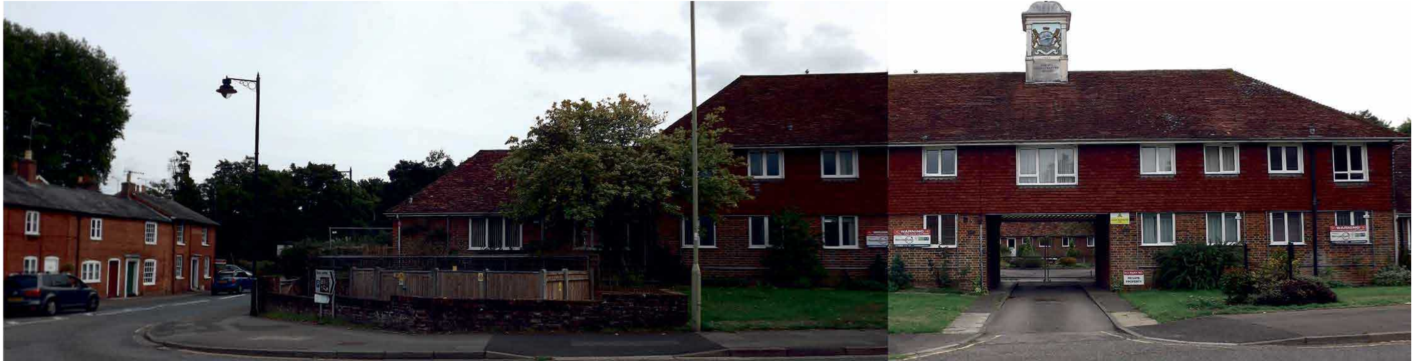
Panoramic of the corner of Palmerston Street and Broadwater Road looking south
