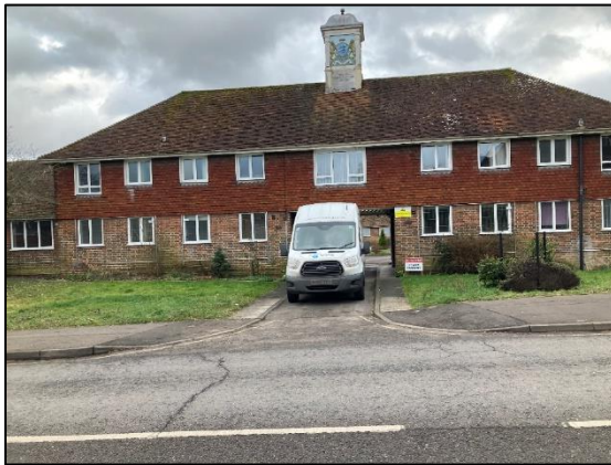
Photograph 1: Existing main site access
