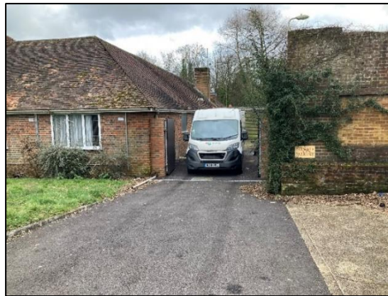
Photograph 16: Proposed Site Access
