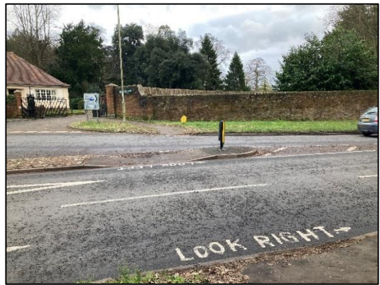
Photograph 11: Refuge Island crossing on Palmerston Street at junction with A27
