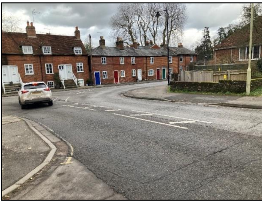
Photograph 10: Informal crossing accompanied by dropped kerbs across Broadwater Road
