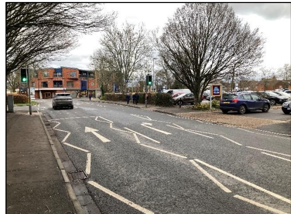
Photograph 7: Signalised pedestrian crossing on Broadwater Road to the west of the site
