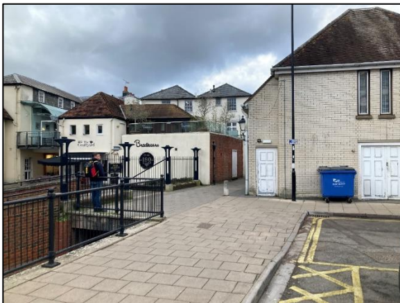
Photograph 12: Footway providing access to High Street from Romsey Bus Station
