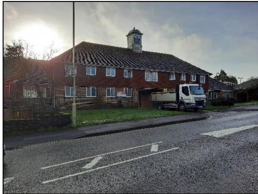
Road Frontage – Broadwater Road
