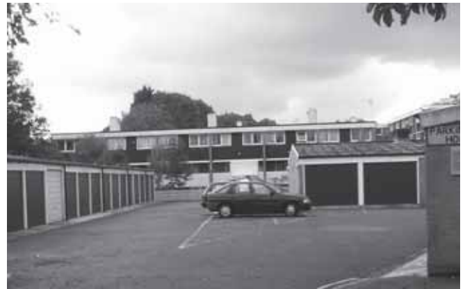
Garages and parking at Broadwater Road
