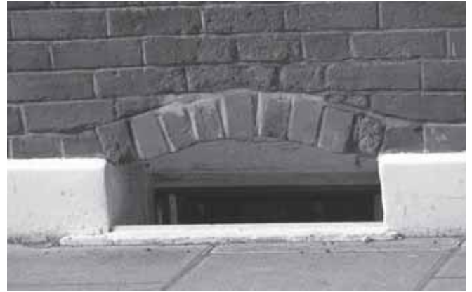
Cellar entrance in Cherville Street
