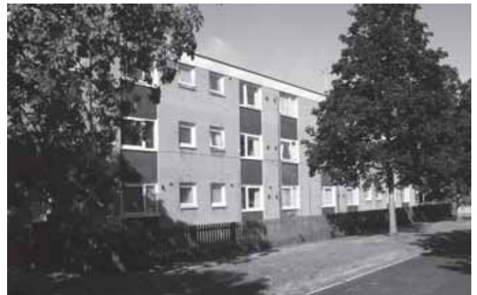
Trees providing a screen in Broadwater Road
