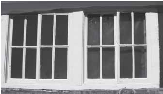
Yorkshire sash window at rear of WH Smith's
