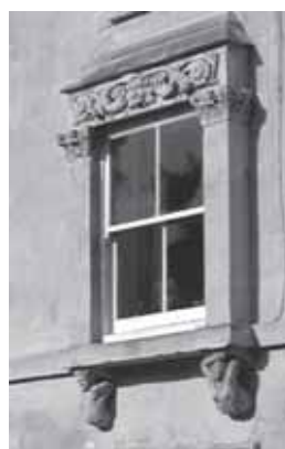
Detail of Bath House, Middlebridge Street
