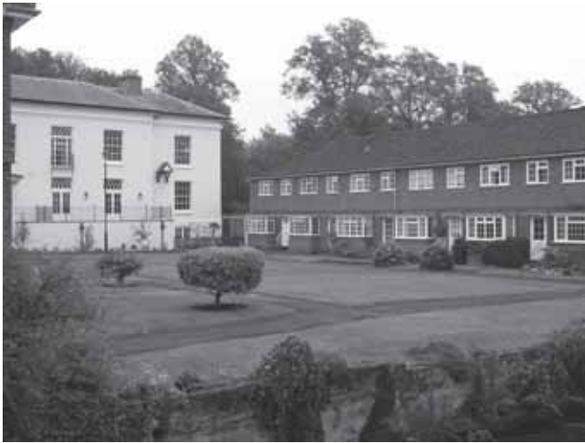
Rivermead House and adjacent terrace
