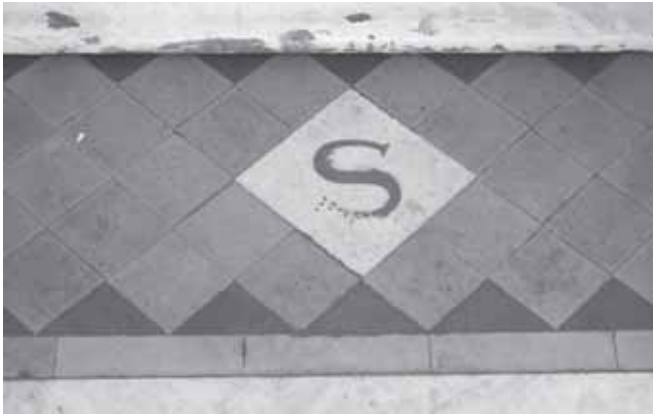
Detail at entrance to shop in The Hundred
