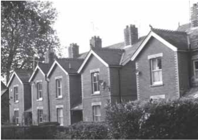
South Front adjacent to By-pass
