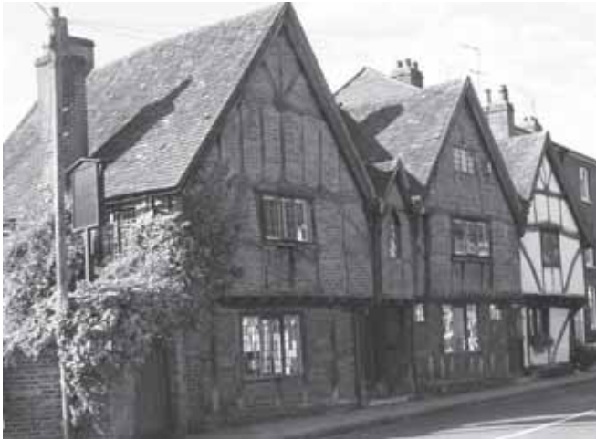
Timber framed building, Palmerston Street
