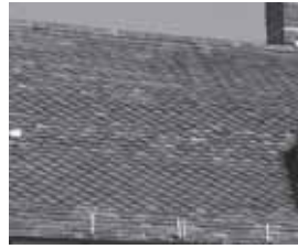
Tiled roof in the old brewery
