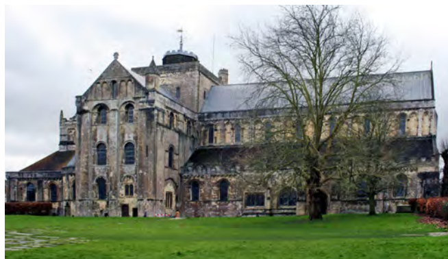
Romsey Abbey, is perhaps the most significant building in the Conservation Area, and one of only three which is Grade I listed, the highest level of designation.
