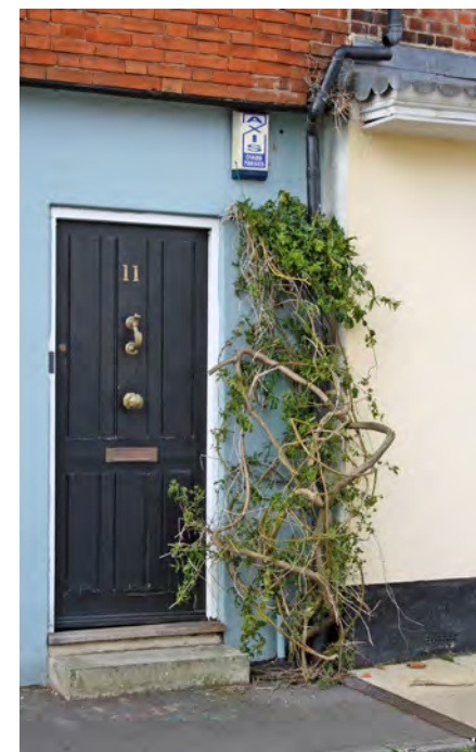
Examples of foliage and algae growth, peeling paintwork and rotting timber all of which are preventable through routine maintenance
