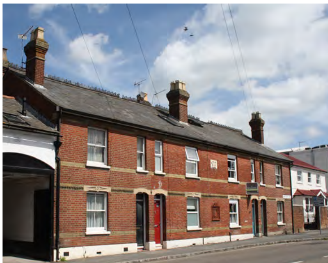
Example of the simple brick detailing present on many buildings in the Conservation Area
