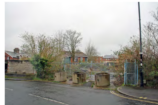
This view from the edge of the Conservation Area into the vacant Strong & Co brewery site demonstrates the detrimental impact it has on the setting of the Conservation Area
