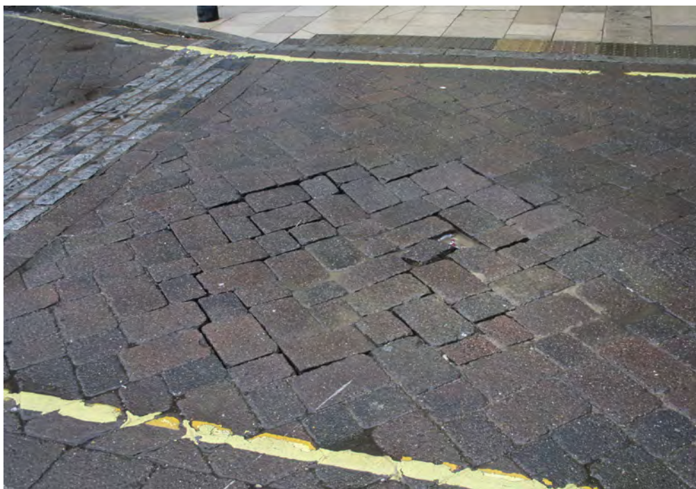
Examples of areas of damaged and patched surface treatments
