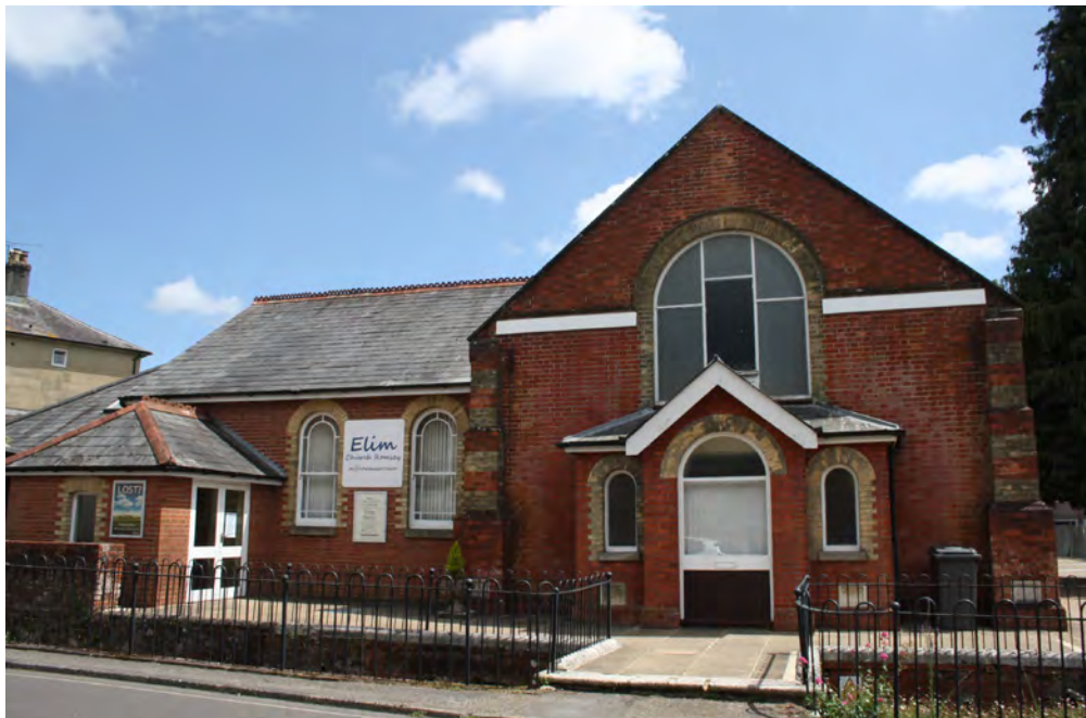
The late-Victorian Primitive Methodist Chapel, now Elim Pentecostal Church, on Middlebridge Street
