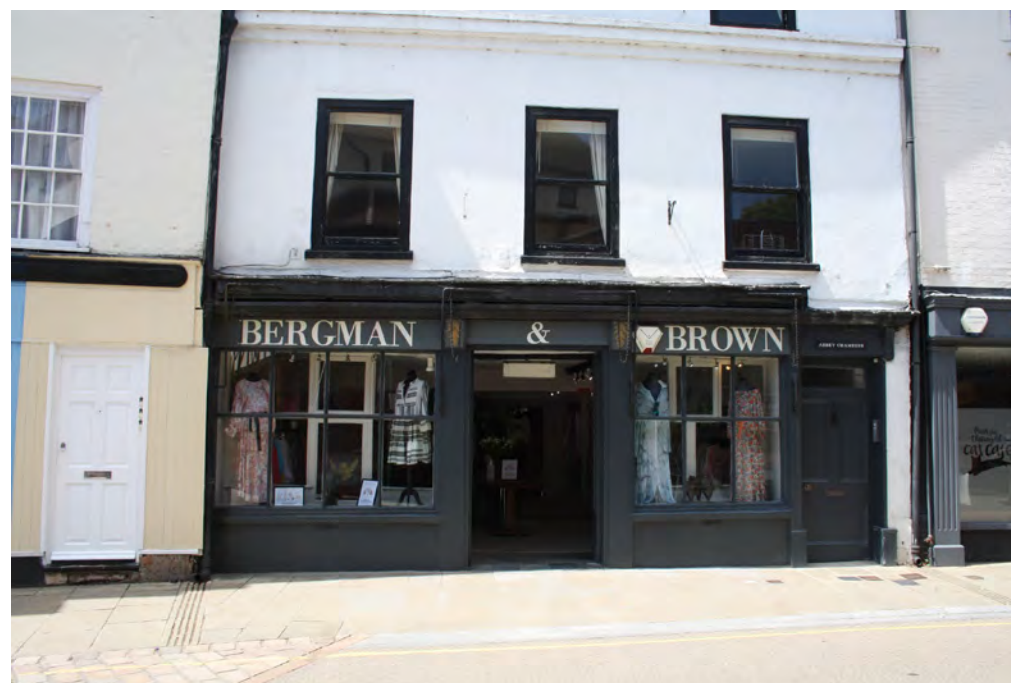
Example of a traditional shopfront in Church Street, containing many historic features such as pilasters, stall risers and fascia board and using timber and glass materials.
