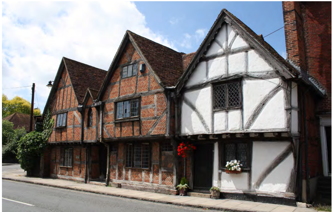
The Manor House in Palmerston Street, a surviving 15th to 16th century timber-frame building with brick infilling
