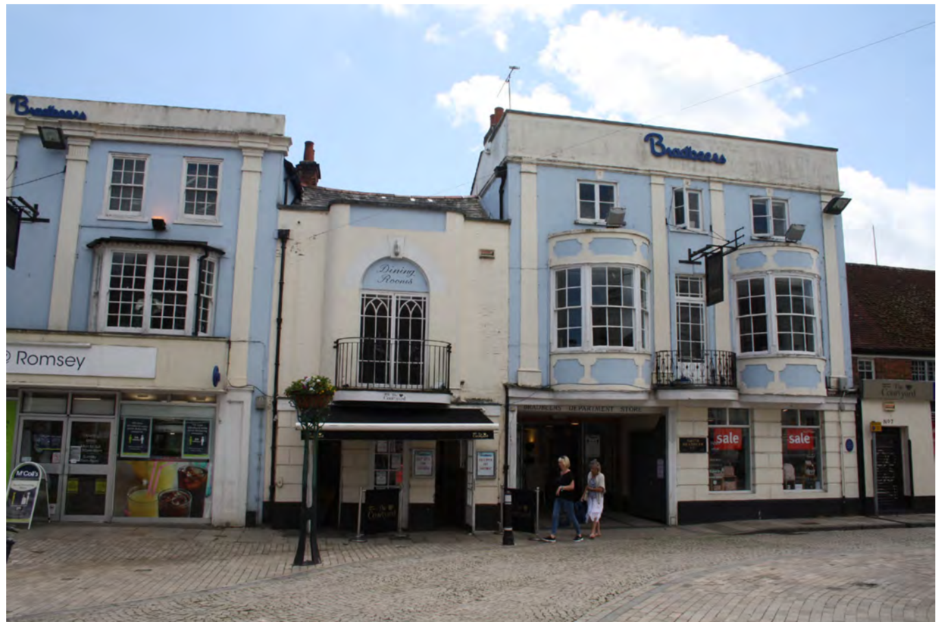
The Dolphin Inn is an 18th century coaching inn now part of Bradbeers department store
