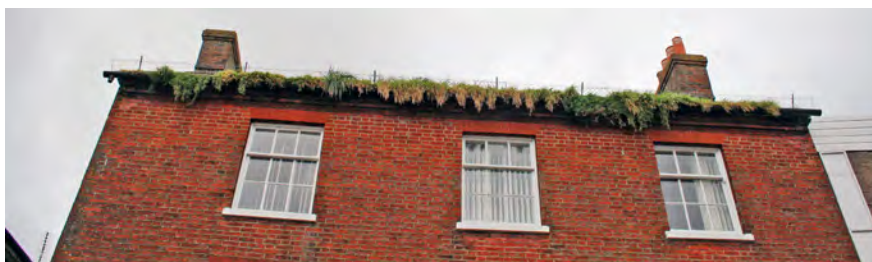
Examples of foliage and algae growth, peeling paintwork and rotting timber all of which are preventable through routine maintenance
