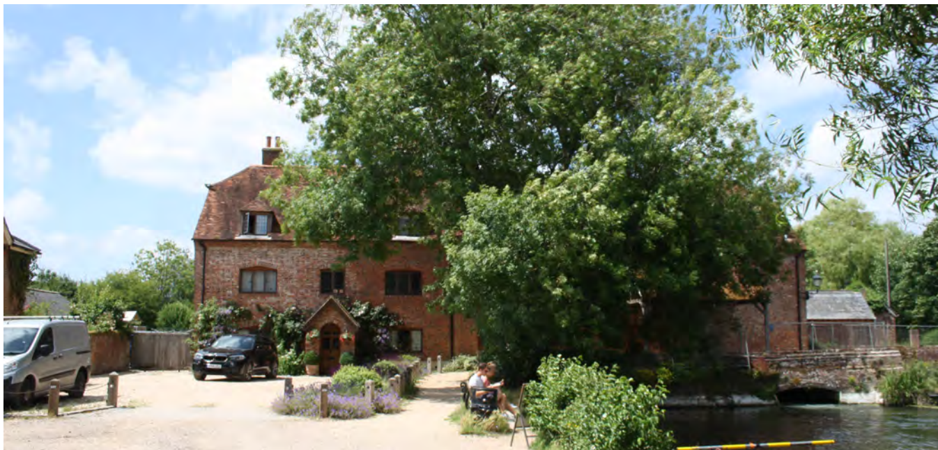
Sadler's Mill, one of Romsey's surviving historic mills located on the main branch of the River Test
