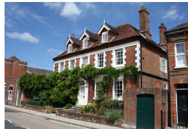
Wykeham House, one of the larger villas on the south side of The Hundred
