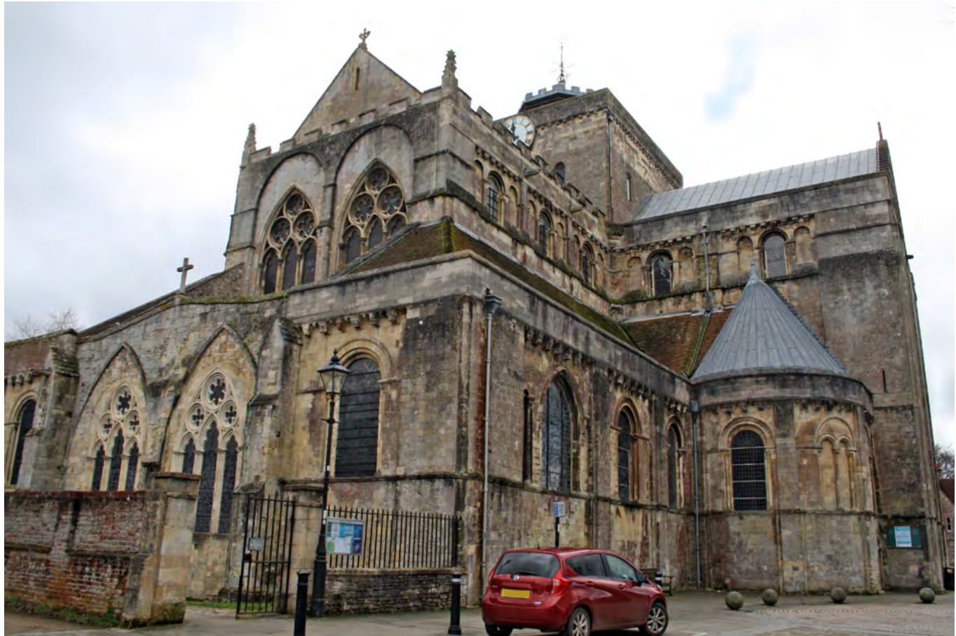
Romsey Abbey, the most significant building in the Conservation Area
