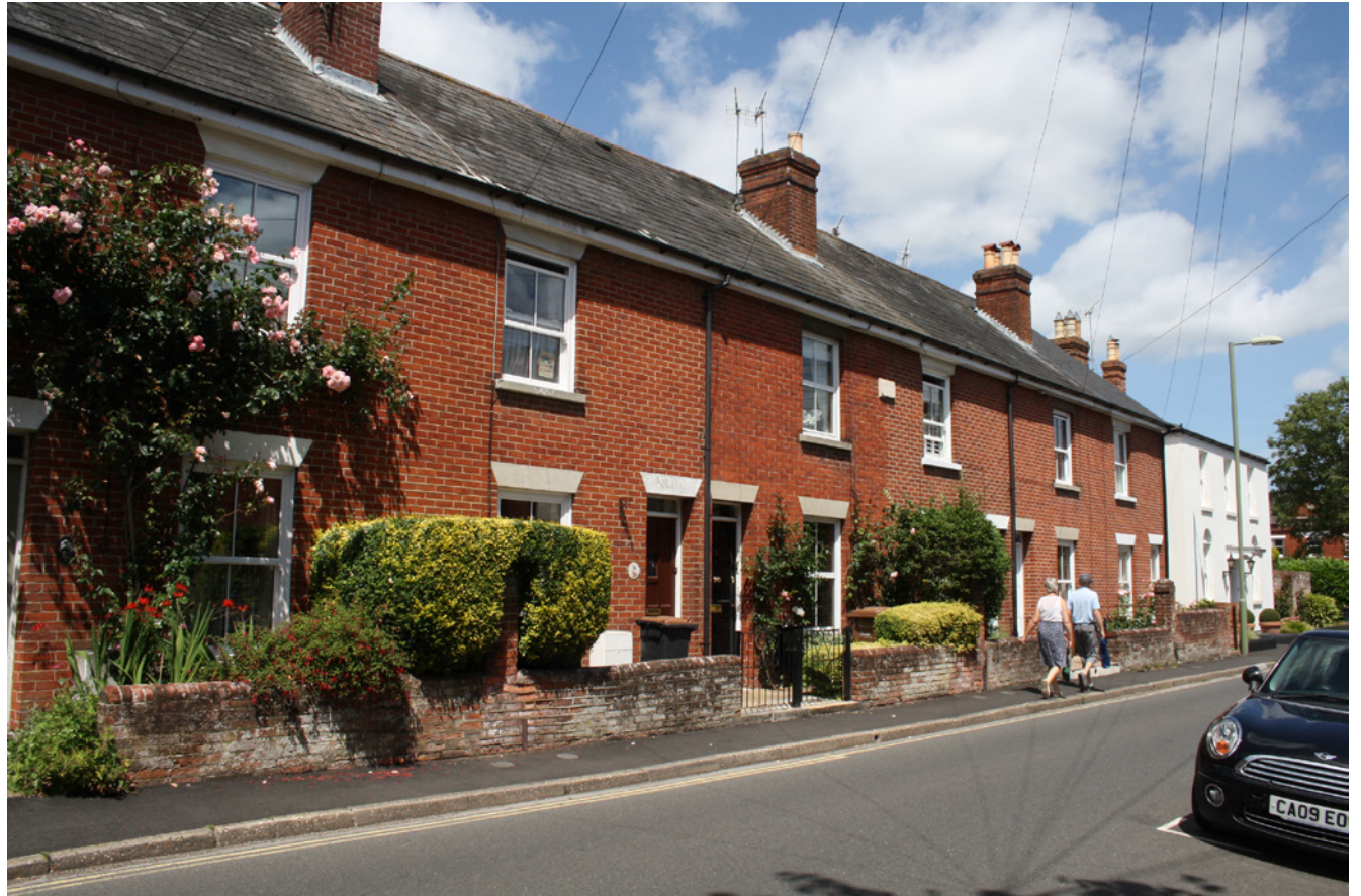
Nos.72-84 Greatbridge Road
