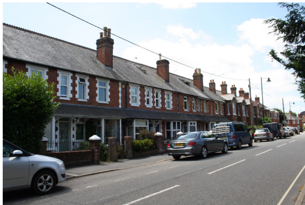
Terraced houses at the west end of Station Road
