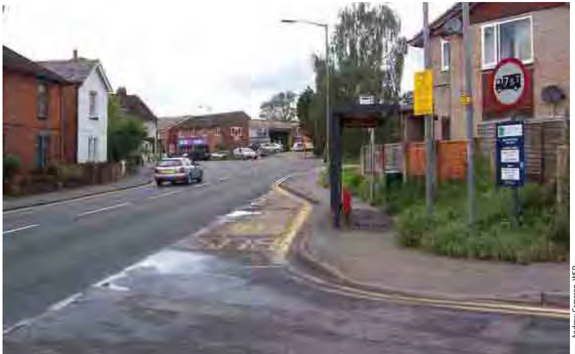
Figure 6.17 The bus lay-by facilitates the free movement of other vehicles, but it is inconvenient for pedestrians.
