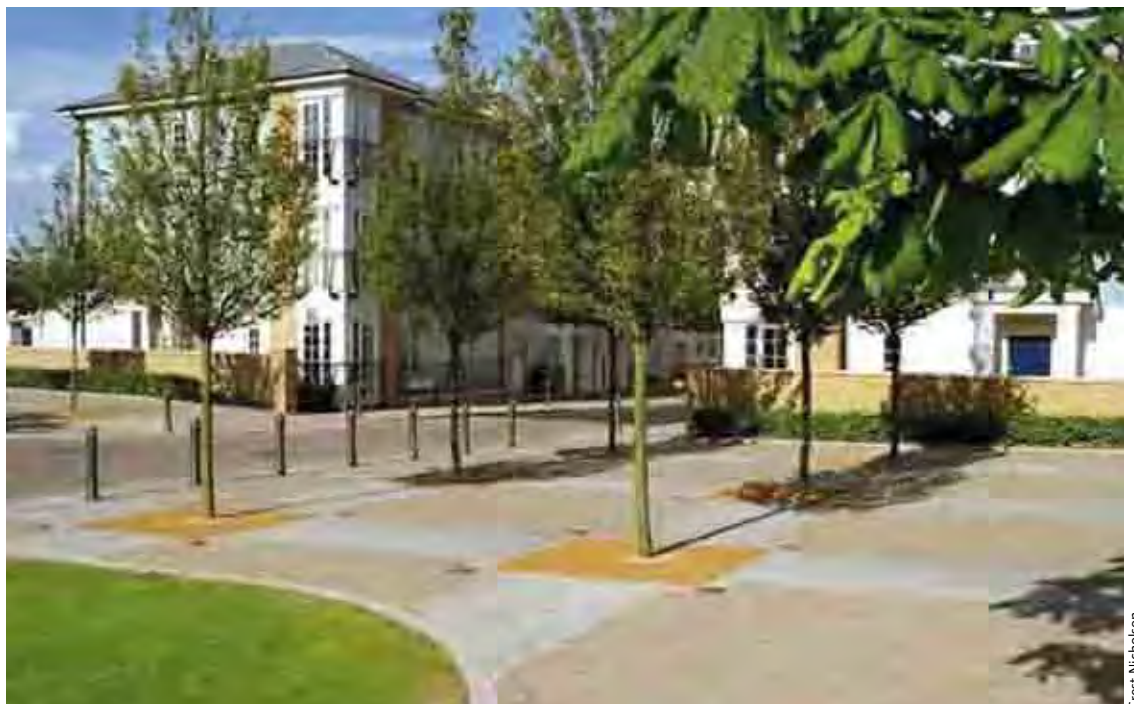
Figure 11.1 The use of good-quality materials achieves a sense of place without leading to excessive maintenance costs.
