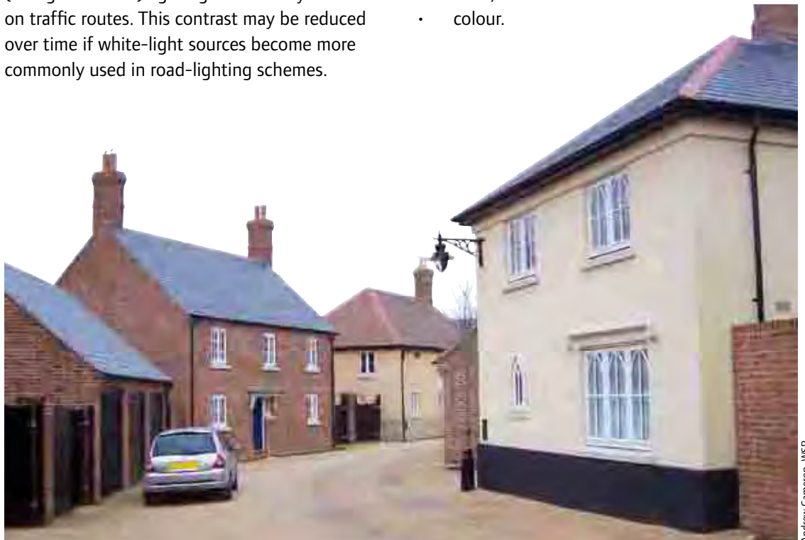
Figure 10.3 Street light mounted on a building.
