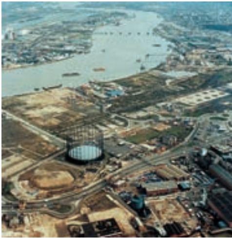
Urban design studies for the Greenwich Peninsula have had to address a wide range of engineering constraints
