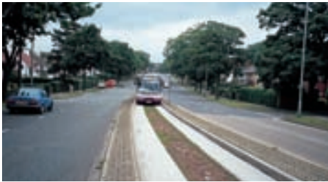
Dedicated busway, Leeds
