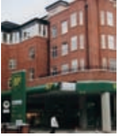
Flats over a garage: where there's a will, there's a way
