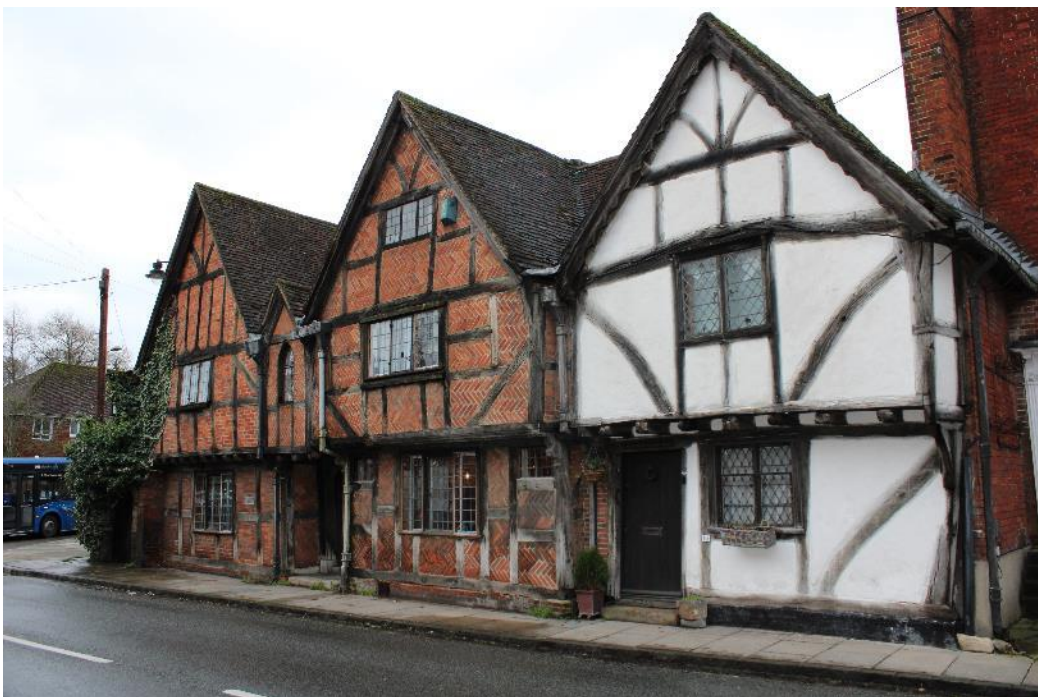
Plate 9: Manor House- 19-21 Palmerston Street
