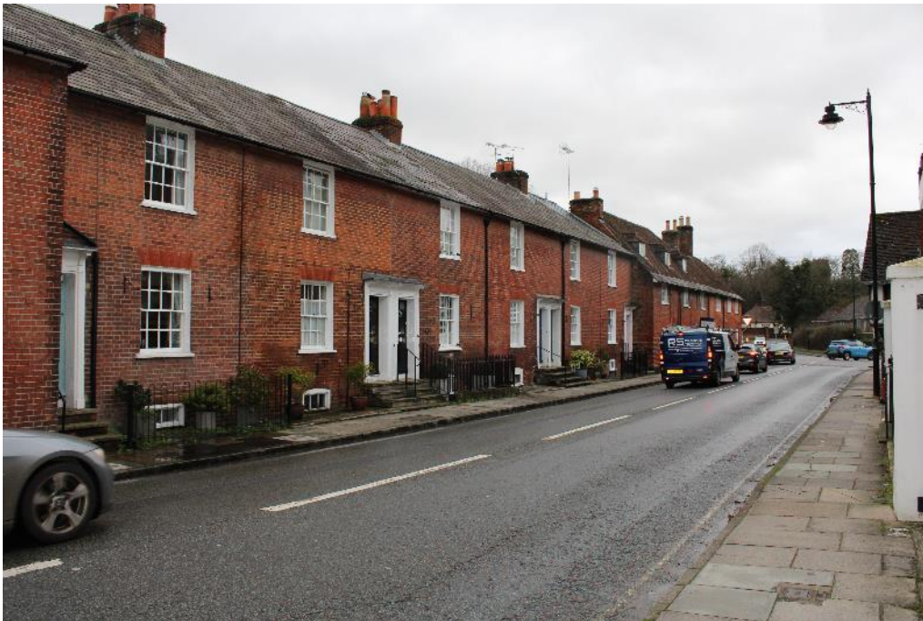
Plate 21: 6-18 and 20-28 Palmerston Street looking southwards to appeal site
