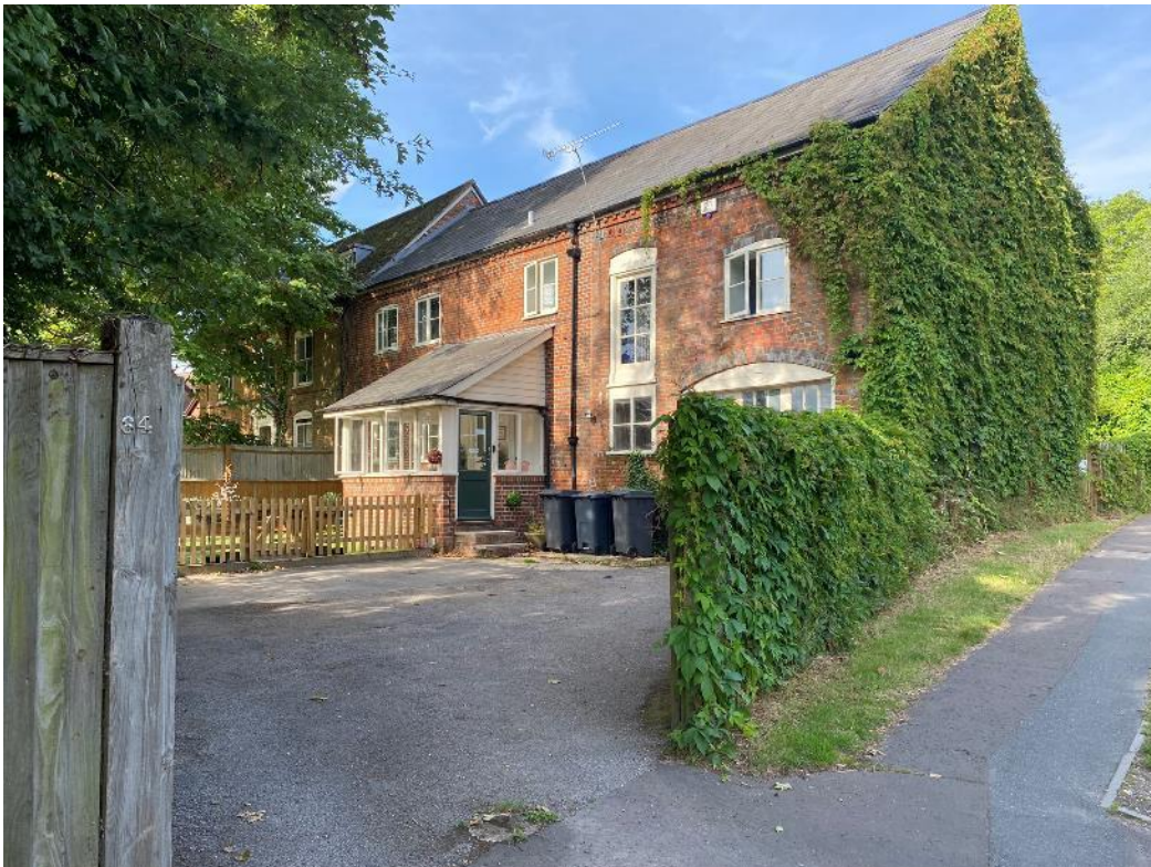
Plate 15: Mill Cottage, 64 Palmerston Street
