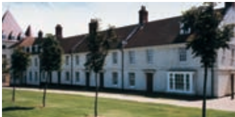
A busy road is addressed positively in Poundbury, Dorset, with boulevard planting and a strong building frontage
