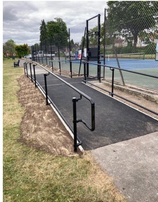
Figure 1: The new accessibility ramp at Vigo Recreation Ground
