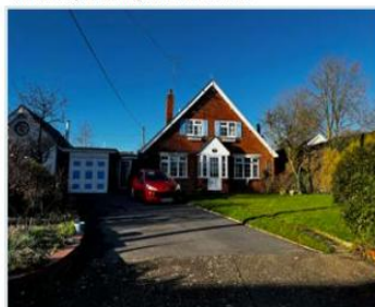
Figure 30: Positive example of a side extension that is appropriately scaled and mimics the original property's roofline, use of material and colour scheme.
