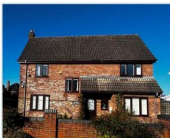
Figure 29: Front porch extension that is in-keeping with the use of material and roofline of the original property.
