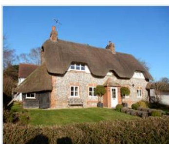
Figure 25: Side extension that is in-keeping with the original property's use of material and appropriately scaled.
