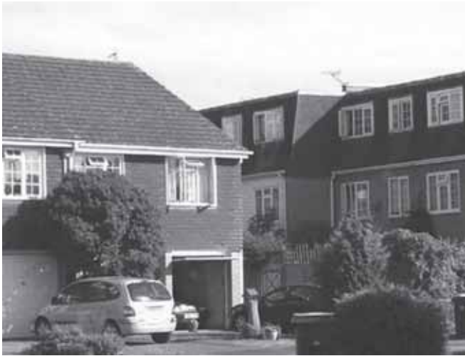
The Thicket showing 2- and 3-storey houses
