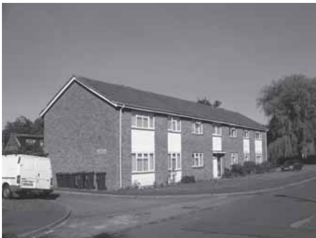
Flats in Symes Road
