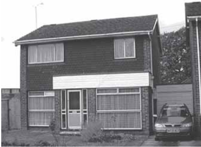
Queens Close reflecting original design
