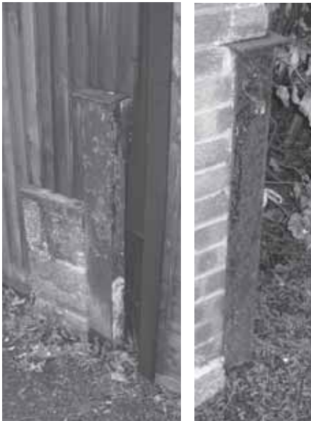
Steel posts from the gateway to the old pig farm
