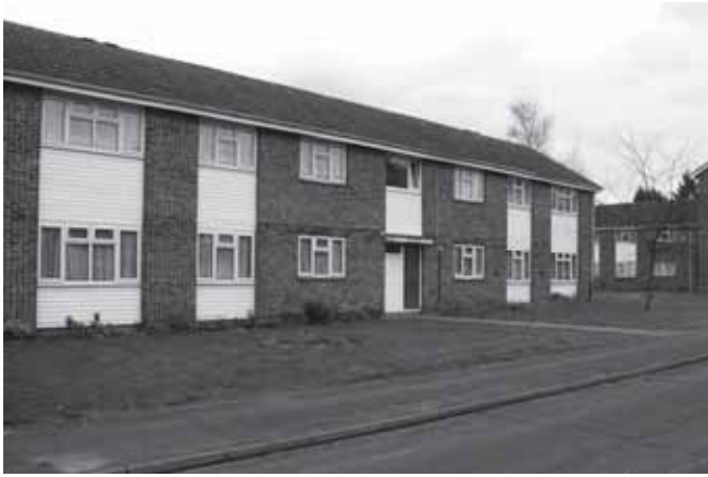
Flats in Chambers Avenue
