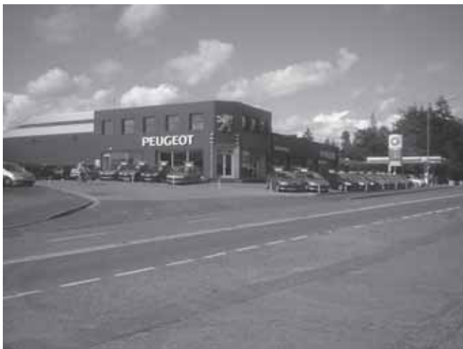
Garage and Convenience Shop
