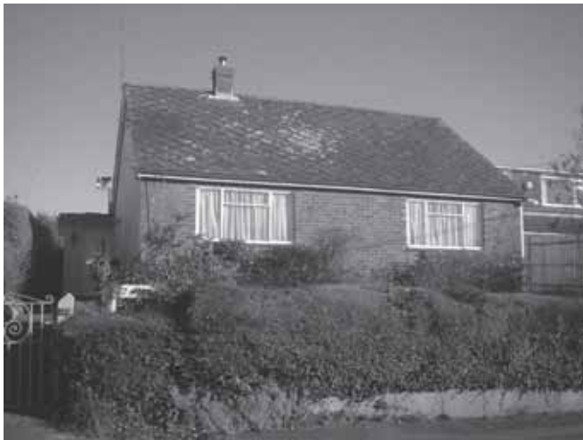
Bungalow with diamond roof tiles
