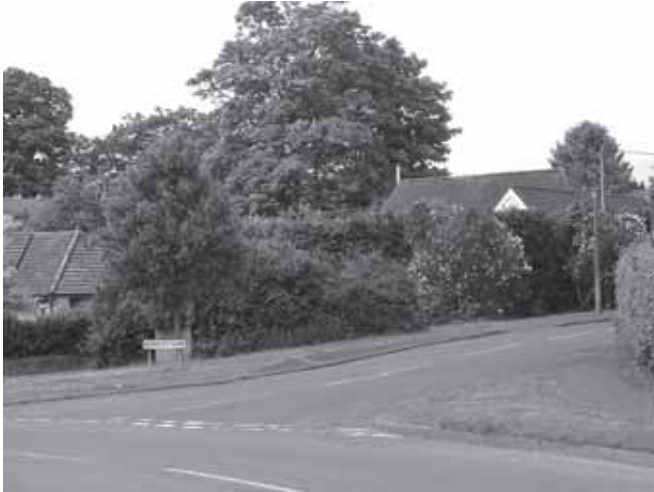
Substation in shrubs, Woodley Lane
