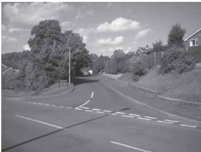
Richmond Lane, looking North East
