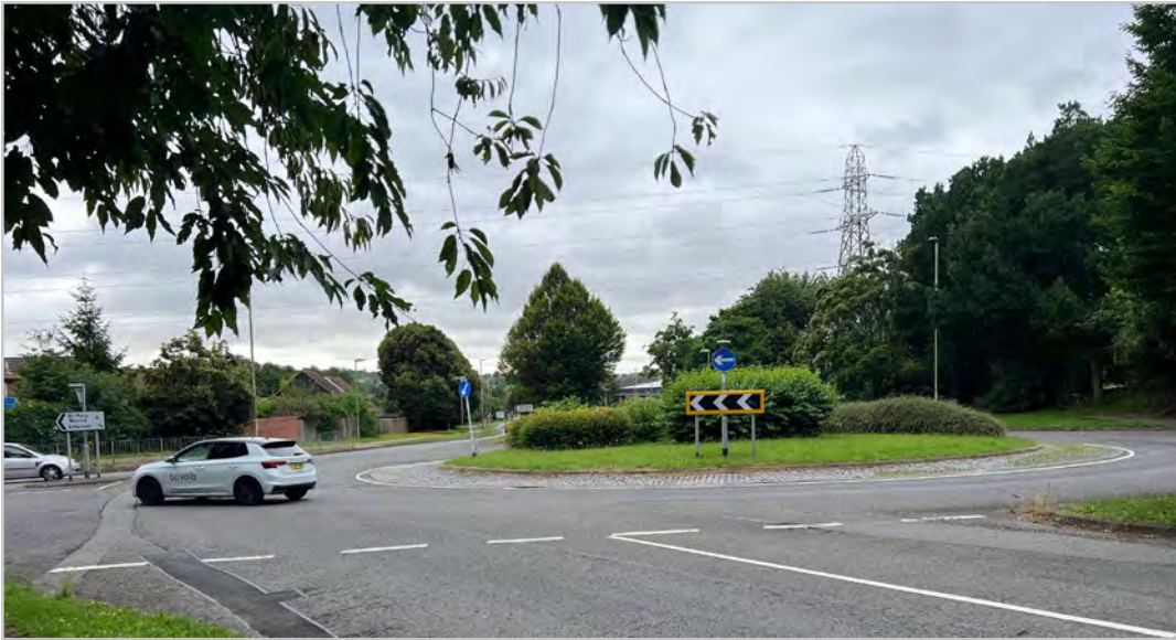
110.1.5 – Smanell Road/Newbury Road roundabout
