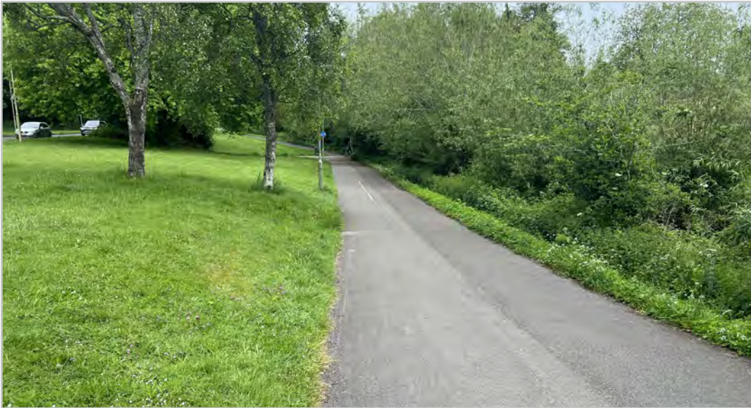
200.1.12 – Shared use facility along Western Avenue
