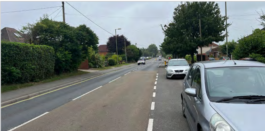
200.1.2 – Weyhill Road conditions east of Weyhill roundabout
