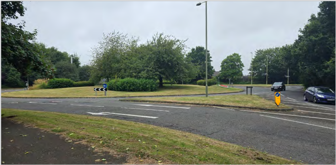
110.1.3 – Roman Way/King Arthurs Way/Newbury Road roundabout
