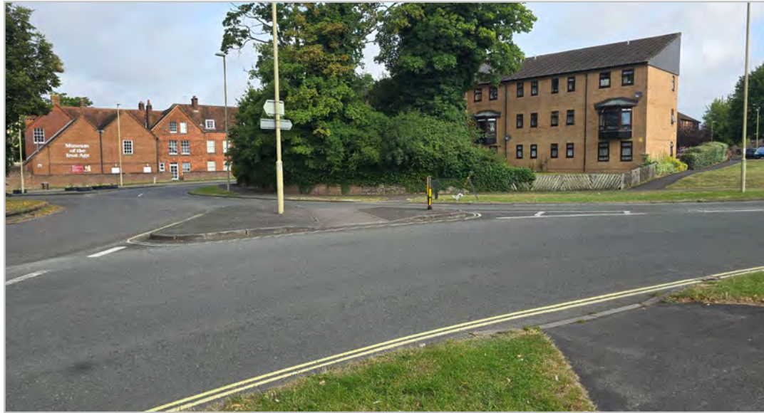
200.3.1 – Vigo Road roundabout
