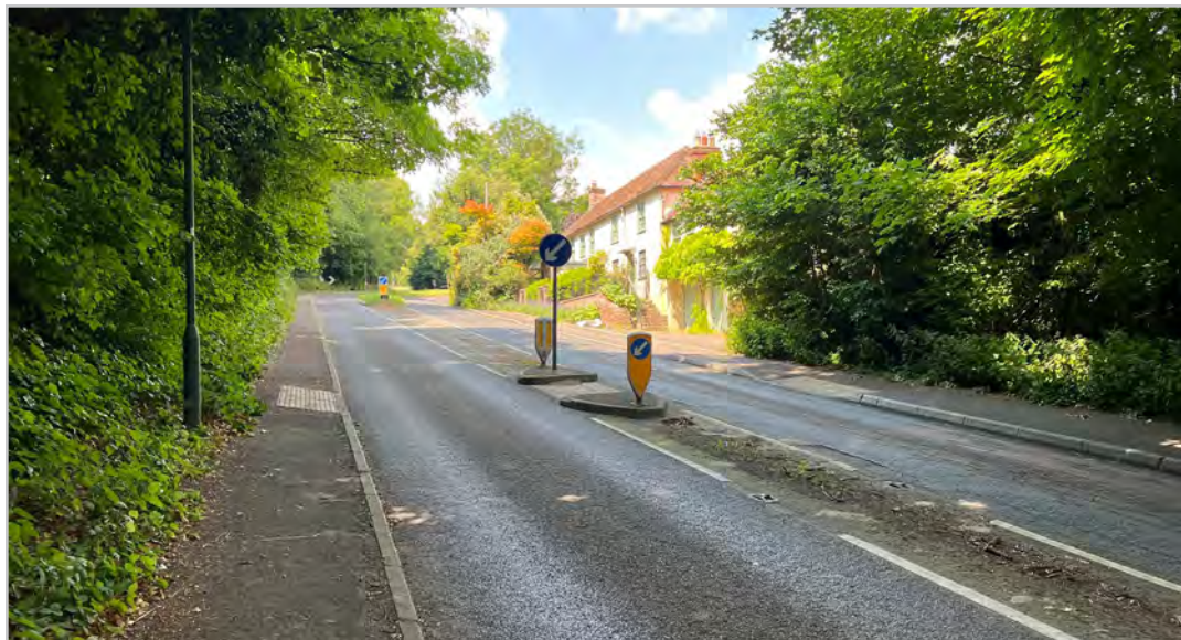
WZ2.1.2 – Uncontrolled crossing on Salisbury Hill
