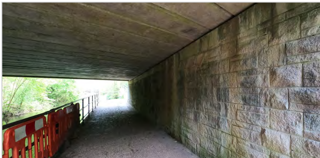
WR1.1.8 – Pedestrian underpass beneath Northern Avenue
