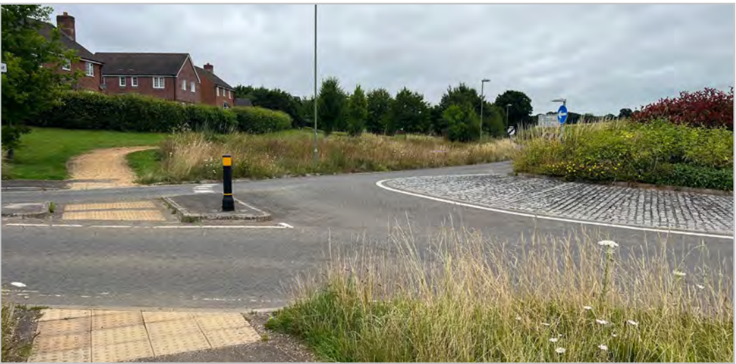
220.2.2 – Crossing Point over Smannell Road/Finkley Road
