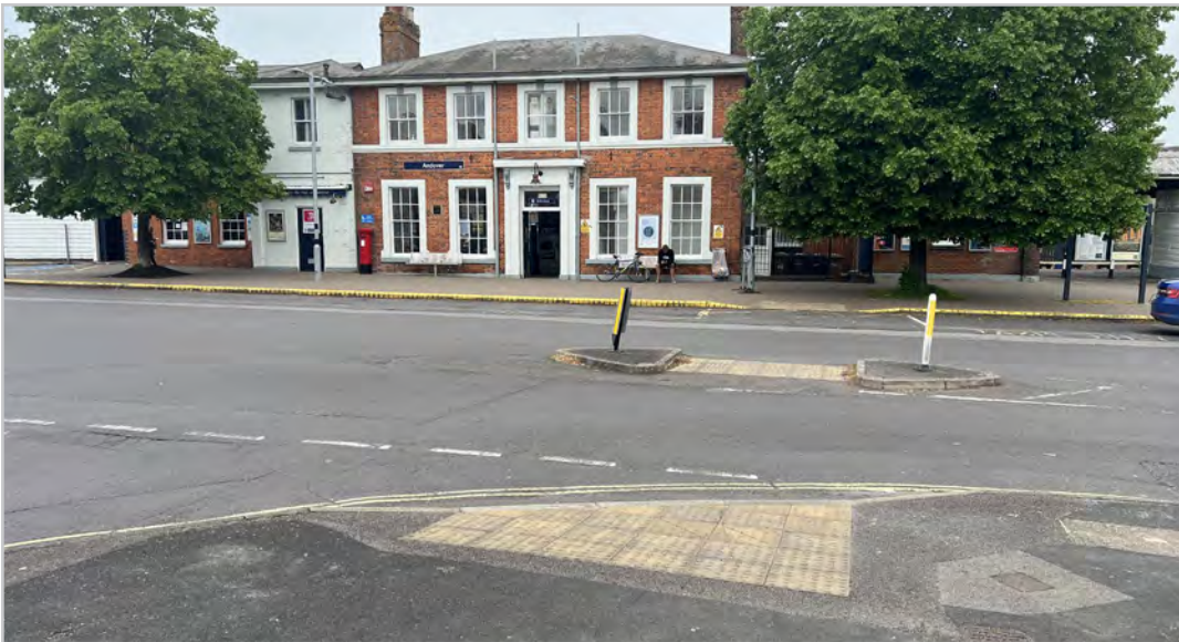
200.1.7 – Andover railway station entrance
