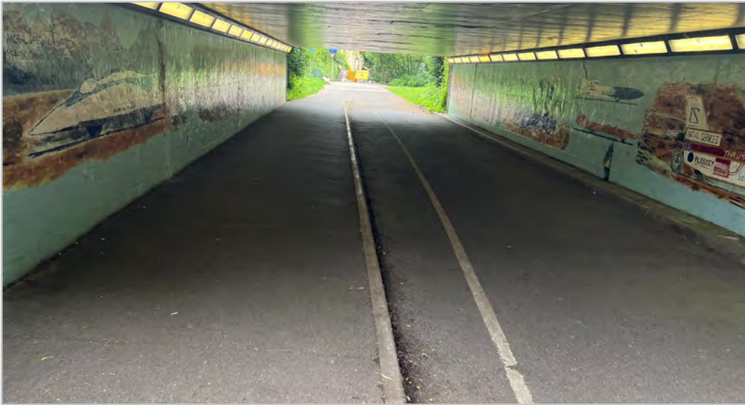
200.1.11 – Underpass beneath Western Avenue
