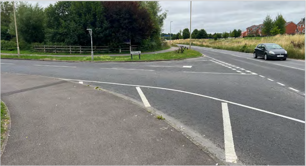
220.1.4 – Junction of Icknield Way and Smannell Road
