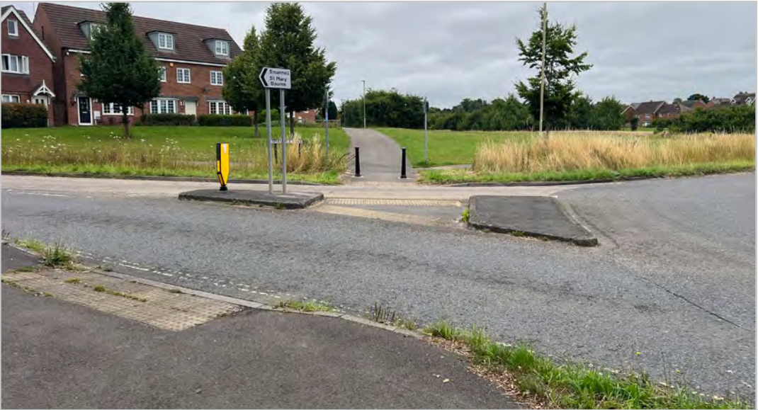
220.1.5 – Crossing over Smannell Road
