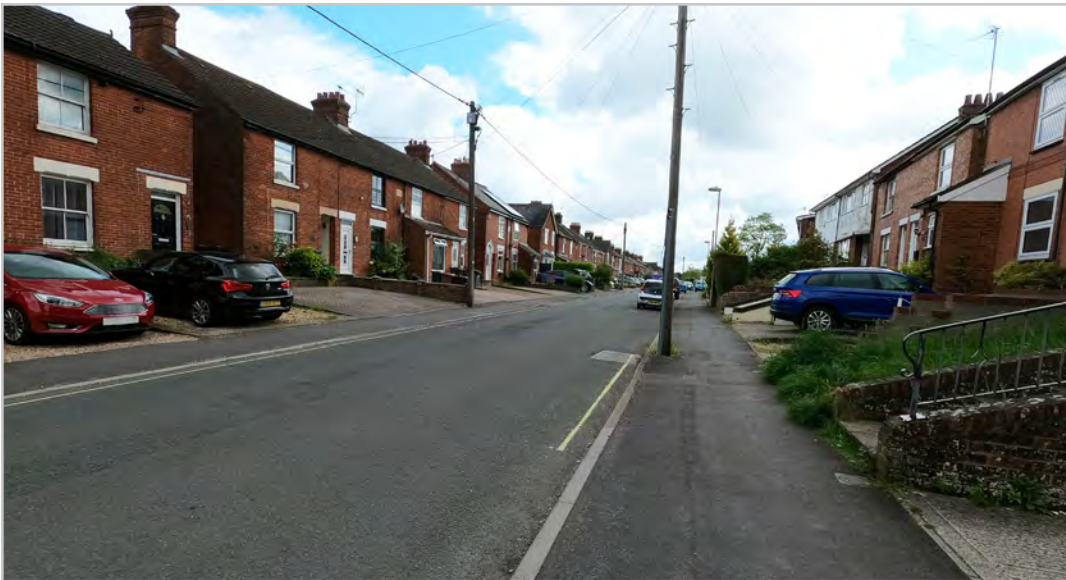
WR1.3.4 – Vigo Road pavement
