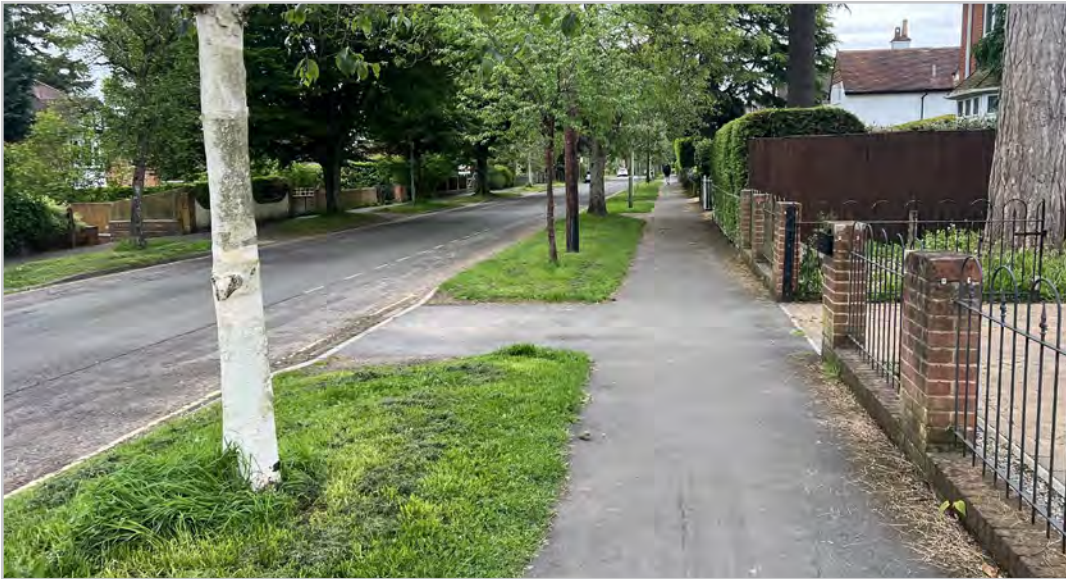
200.1.9 – Bishops Way footway
