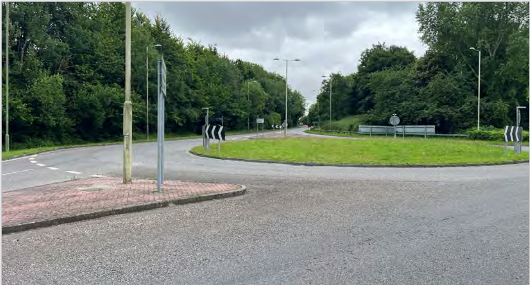
110.1.2 – Saxon Way/Newbury Road roundabout
