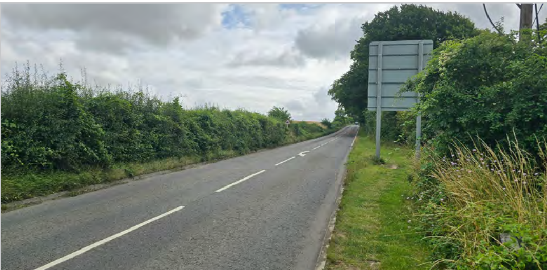
230.1.4 – Conditions of London Road beyond Picket twenty roundabout
