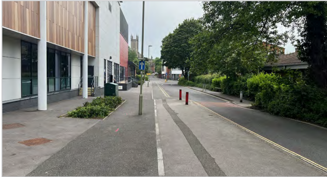
200.2.1 – Shared use facility along West Street
