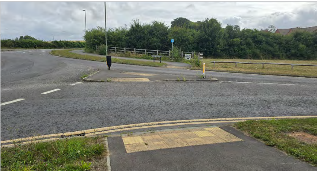
230.1.3 – Picket Twenty roundabout
