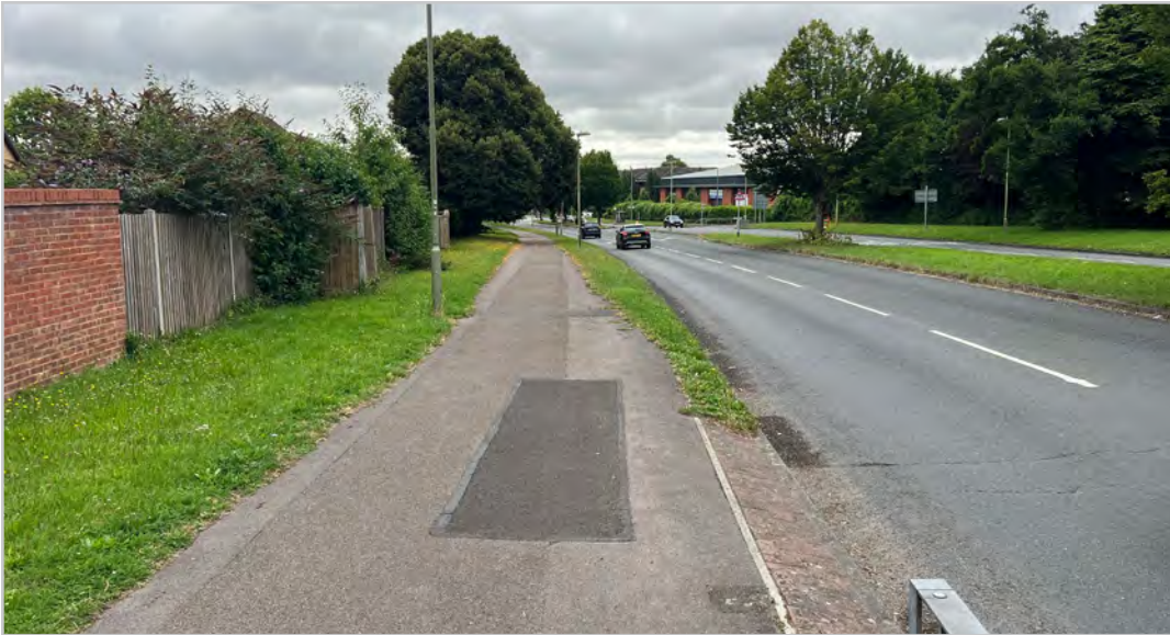
110.1.6 – Newbury Road near railway bridge
