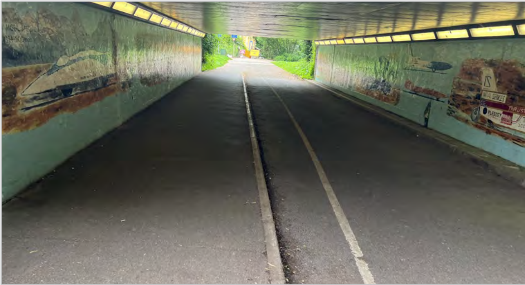
WR1.8.1 – Photo of Western Avenue Underpass
