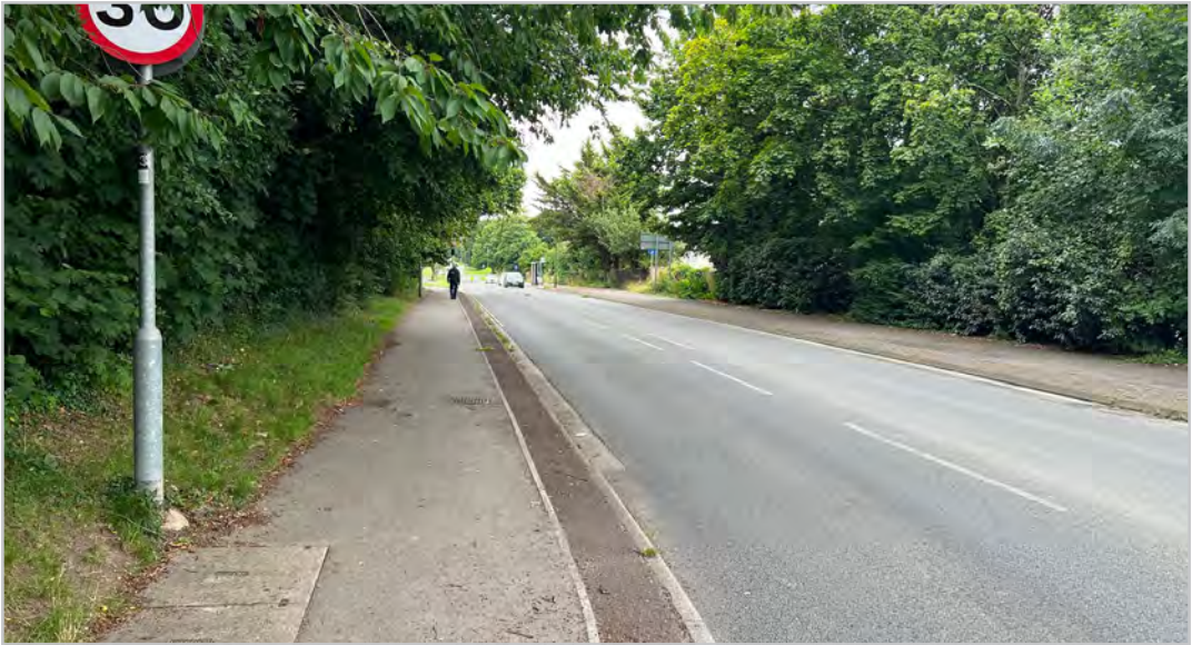
220.1.1 – Smannell Road footway
