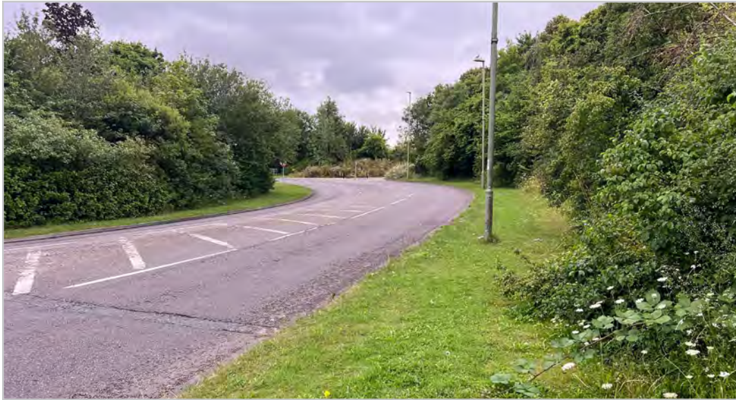
100.1.5 – Redon Way conditions
