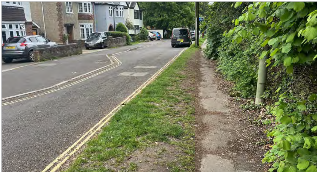
200.1.10 – Junction Road footway
