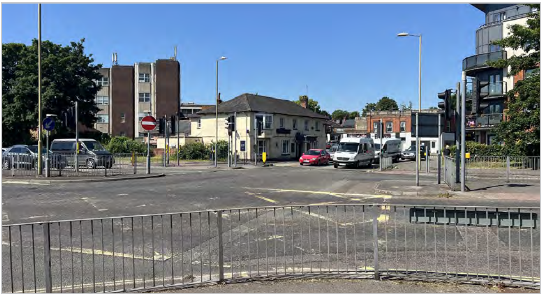
WR1.6.2 – Crossing over Western Avenue
