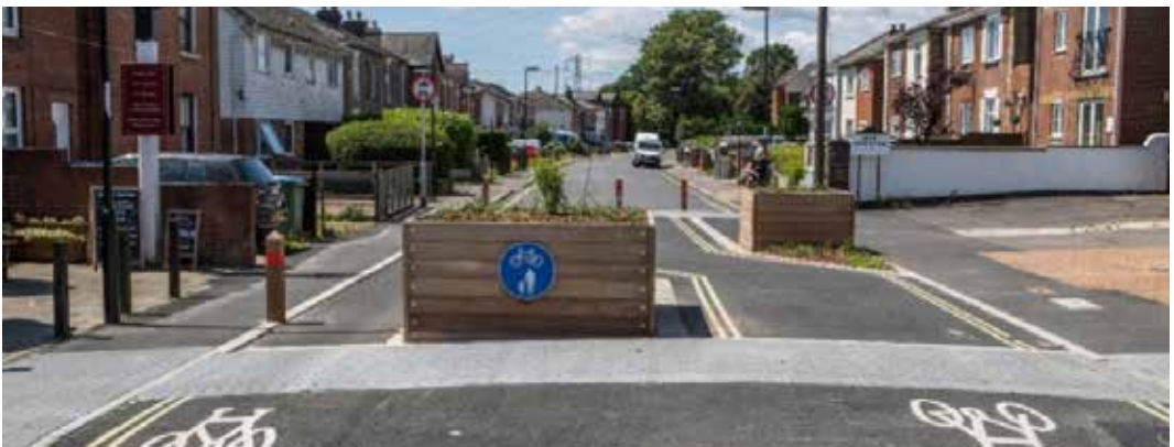
Point closure – SCN 1 Western Cycle Freeway, Southampton
