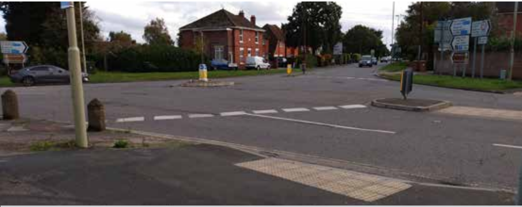
Z1.2.1 Winchester Road roundabout
