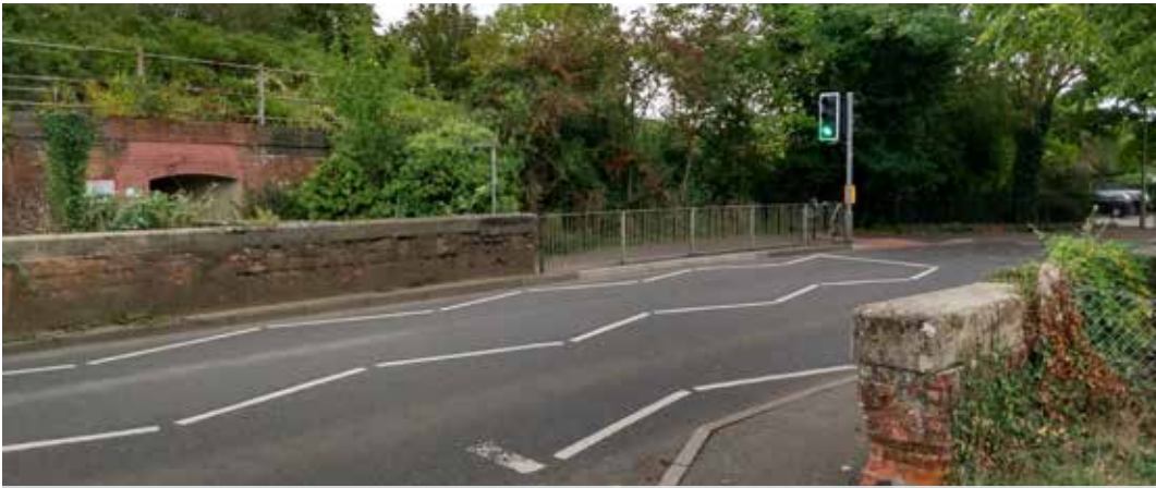
282.2.4 A3057 Railway Track Underpass
