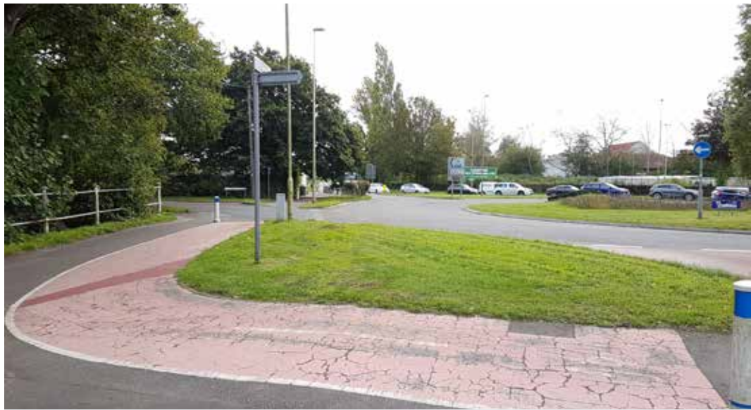
330.1.6 A3090/A27/Knatchbull Close roundabout
