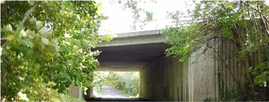
263.1.1 Upton Lane M271 underpass
