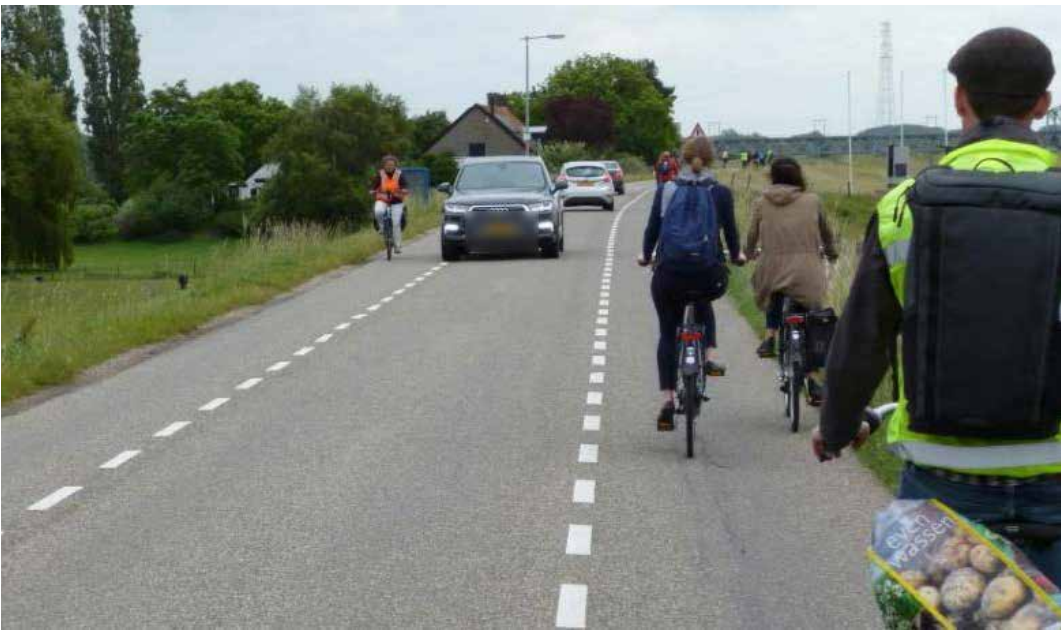
Dutch style street Street without a centre line encourages slower vehicle speeds and helps create a shared street environment.
