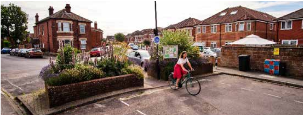
Example of a point closure – Alma Road, Southampton. Photo credit: J. Bewley – Sustrans
