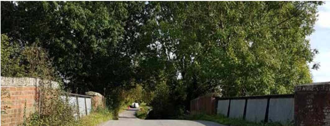
263.1.1 Upton Lane rail bridge
