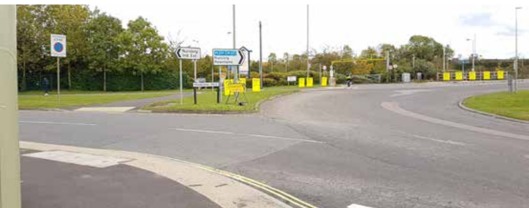
330.4.3 Andes Way/Brownhill Way roundabout
