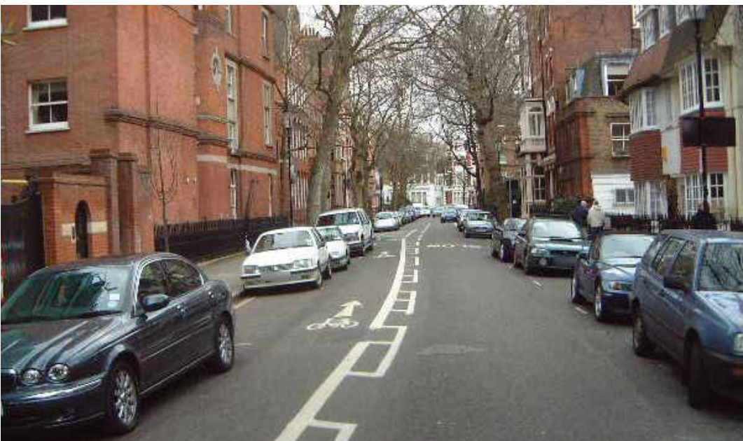
Contraflow cycle lane Mandatory cycle lane that allows cyclists to travel opposite the flow of vehicle traffic, allowing for greater permeability of the cycle network.
