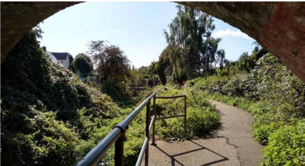
331.1.1 Path under railway tunnel
