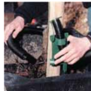
▲ Fitting a Tree Watering System
