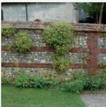
Detail of brick and flint churchyard wall
