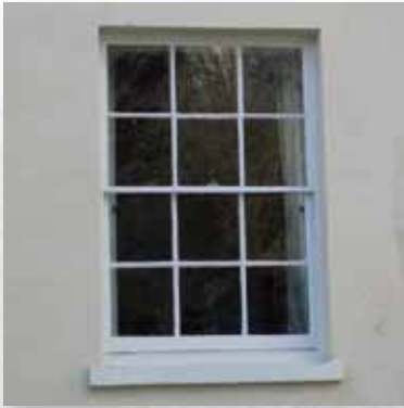
The Old Vicarage sash window
