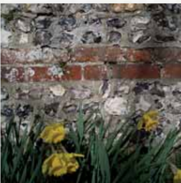
Church flint and brick wall
