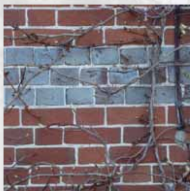
The Old Plough brickwork detail
