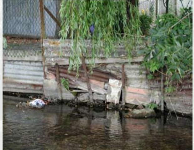
Photo 5: Make-shift revetment constructed from corrugated iron. Revetment like this offers no habitat value and, if washed out, could block downstream culverts and cause flooding.
