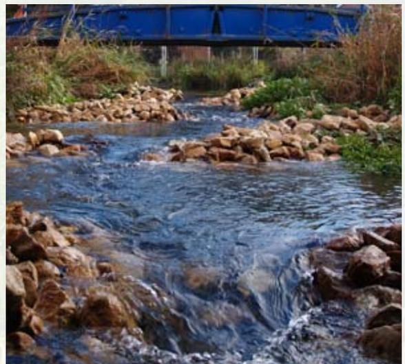
Photo 21: A 'rock-ramp' recently installed during redevelopment beside the river at Anton Mill Road. This structure has replaced a conventional over-shot weir, resulting in improvements to fish passage and reduced flood risk. Its in-built flexibility enables future improvements to be made at low cost.
