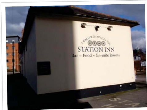
Rear of the Station Inn, Andover
