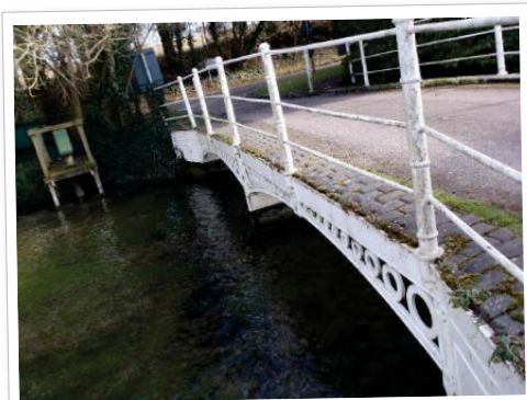
Taskers Iron Bridge
