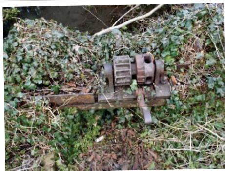
Gearing for a sluice gate
