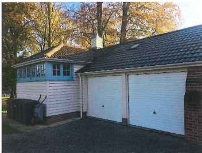
Photo 1: External view of building A
