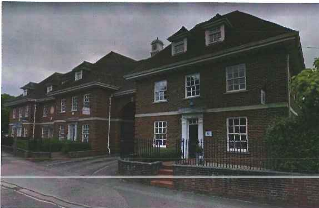
Figure 8b: Eastwood Court Buildings Frontage (Source: Google Maps)
