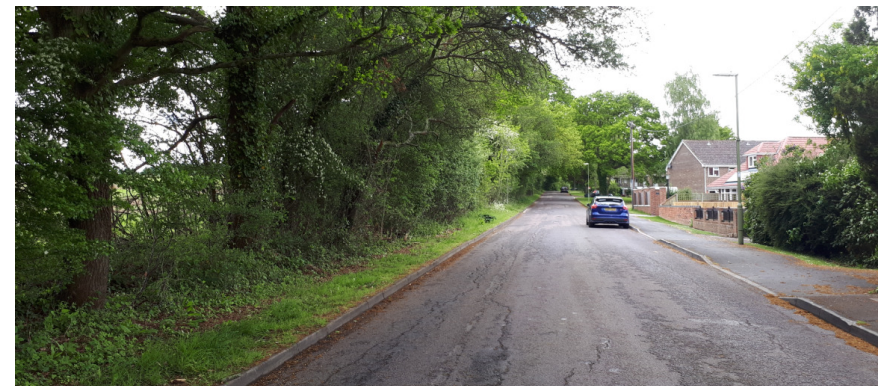
Image 52 (above) Hoe Lane street scene with vegetation
