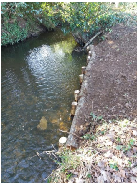
River bank revetment works
